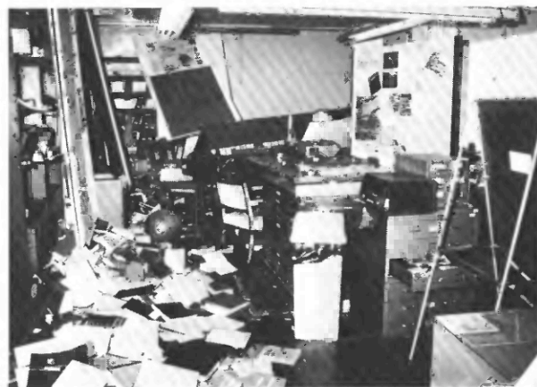
FIGURE 44.11.—Main meeting room and library at Hawaiian Volcano Observatory after 1983 earthquake. Bookcases were torn from back wall and fell onto table; storage cabinets were moved as much as 0.5 m. Preearthquake location of cabinets is documented by dust marks on floor behind and to right of plastic waste bin. Smoked-drum seismographs (obscured by easel) located under windows to right were temporarily out of order because their drive mechanisms jammed. Photograph by J.D. Griggs.
