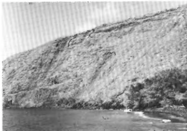
FIGURE 44.32.—Narrow chutes (outlined) formed at time of November 1983 earthquake by landslides from steep slopes surrounding Kealakekua Bay, west coast, Island of Hawaii. Rock falls (rf) occurred on lower, steeper slopes. View northwestward.
