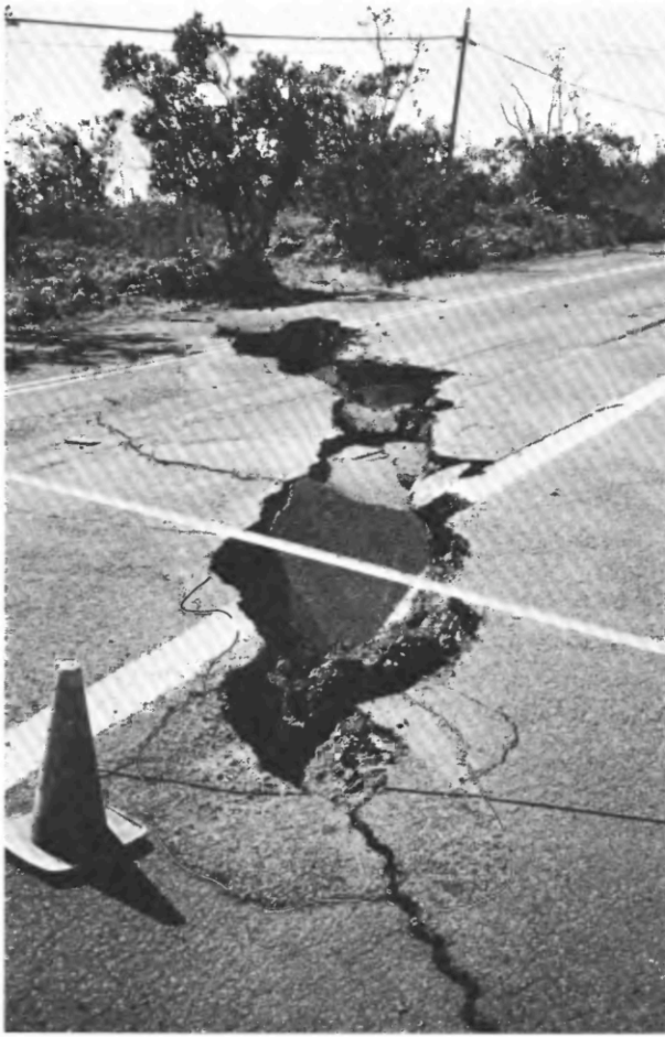
FIGURE 44.21.—Section of Crater Rim Drive at eastern entrance to Kilauea Military Camp that collapsed in November 1983 earthquake along a system of cracks trending at az 60°. Earthquake shaking caused subsurface material to settle, thus undermining road. Note pavement patch from repair of earlier failure at same place.
