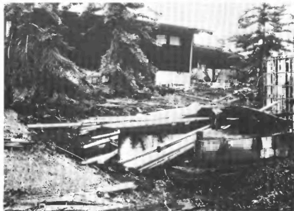
FIGURE 44.13.—Water tanks in Volcano affected by 1983 earthquake. Most water tanks here were constructed like one standing at right rear. Tank in foreground has collapsed, while other appears little damaged although displaced southwestward 0.7 m. This difference in response to earthquake may be because of a difference in water level in tanks at time of earthquake, or because of a difference in age or condition of tanks. Photograph by E.T. Endo.
