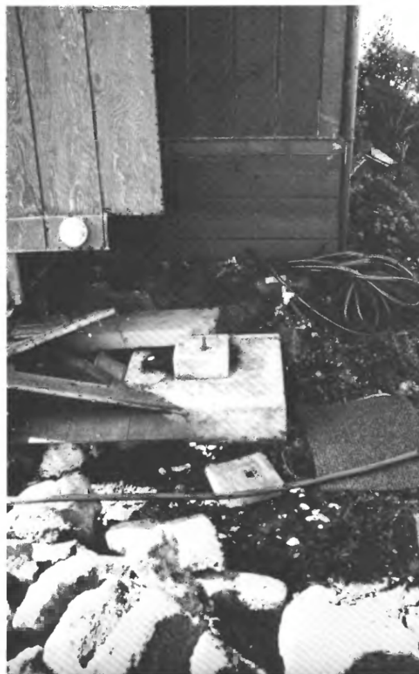
FIGURE 44.9.—North corner pier of damaged two-story frame house in Volcano Golf and Country Club Subdivision. Although house is now 1.2 m southwest of its foundation, rebar protruding through piers is still straight. Termite shield from atop pier can be seen on ground. House subfloor was originally 1 m above ground, but most supporting posts collapsed.
