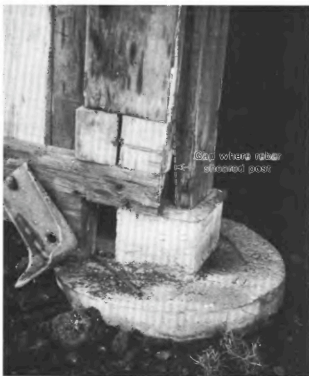
FIGURE 44.12.—Barnlike three-story-high frame house in Puna District that was moved off its foundation about 0.3 m toward northeast in 1983 earthquake. A , View of house showing position of one of sheared support posts (circled). B , Close-up of footing circled in A . The 14-cm by 14-cm wooden post was sheared by rebar that extended from base of footing upward into post as much as 11 cm; most other posts supporting upper story were similarly sheared. House has been replaced on piers.
