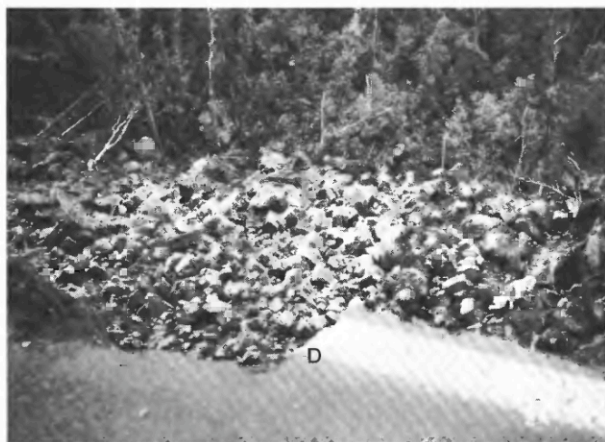
FIGURE 44.24.—Details of failure of Waldron Ledge landslide. Labelled points (A, B, C, D) are same as in figure 44.23. A , View southeast at head scarp of landslide and of parallel graben on other side of road. Headwall scarp was approximately 14 m high and 30 m long; landslide removed 11-m-wide section of road and trail. B , View downward from road of jumbled mass of rock resulting from disintegration of slide block; mass did not travel far from base of cliff.
