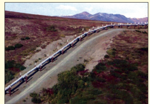
Figure 4. Ground photograph of the Trans-Alaska Pipeline and parallel access road constructed on ice-rich permafrost. The pipeline is constructed on elevated thermopiles to dissipate heat and prevent thawing of permafrost.
