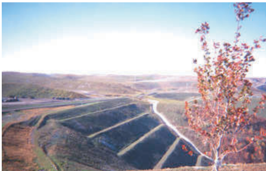
Figure 16. Photograph showing view of excess-spoil fill, or valley fill, in the Samples Mine, Boone and Kanawha Counties, W. Va. The valley fill is stabilized, terraced, and seeded. Photograph by Susan J. Tewalt.
