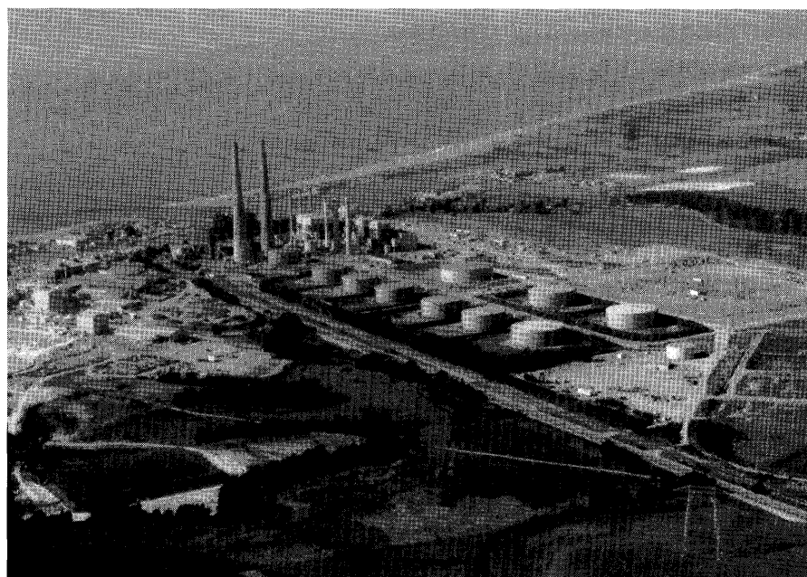
Figure 3.—Pacific Gas & Electric Co. powerplant at Moss Landing (see fig. 2 for location). Moss Landing spit and Moss Landing State Beach are visible in background.
