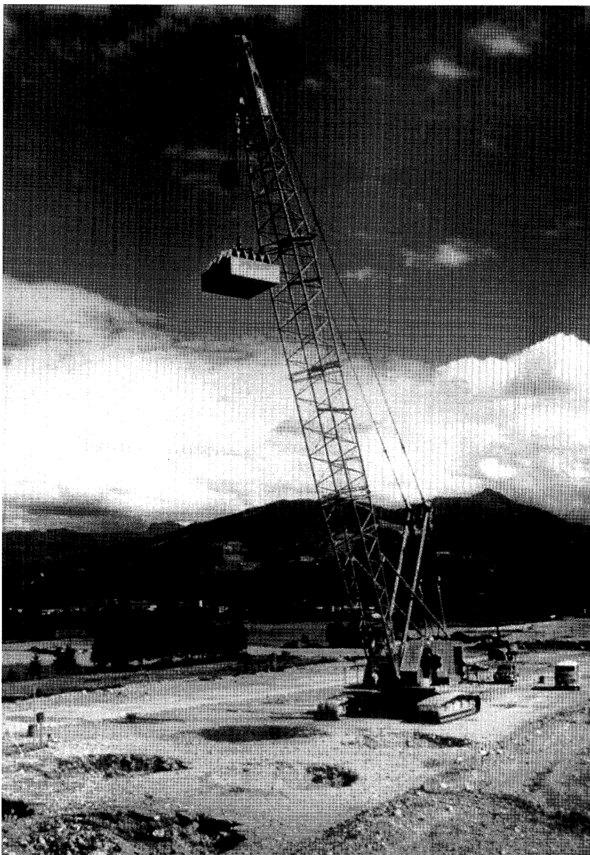
Figure 3.—Dynamic deep compaction in operation.
