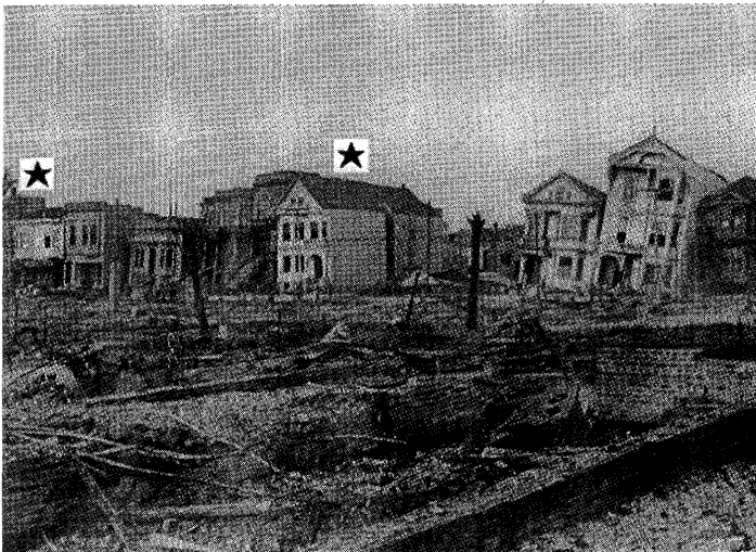
Figure 13.—Buildings on east side of South Van Ness Avenue between 17th and 18th Streets after 1906 San Francisco earthquake and fire. Stars denote structures still standing in 1993. Two buildings to left of center sustained cripplewall failure and were shifted to left (northward) off their foundations. As a result of these failures, they are tilted to right and away from street. Rubble from another building that collapsed into an adjacent vacant lot is visible in center. View from Capp and 18th Streets (see fig. 9 for location).
