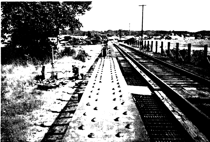
Figure 17.—Test site CSU 48 (fig. 16) at Southern Pacific Railroad Bridge study site (fig. 7).
