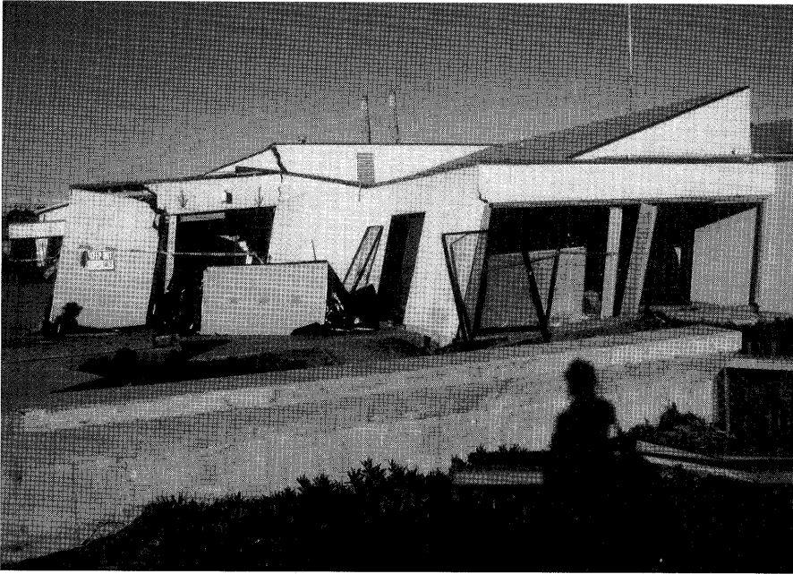
Figure 12.—Racking of director's office at southwest corner of Moss Landing Marine Laboratory (fig. 11).
