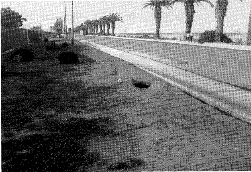
Figure 5.—Sand boil on east side of Treasure Island at locality 5 (fig. 4).
