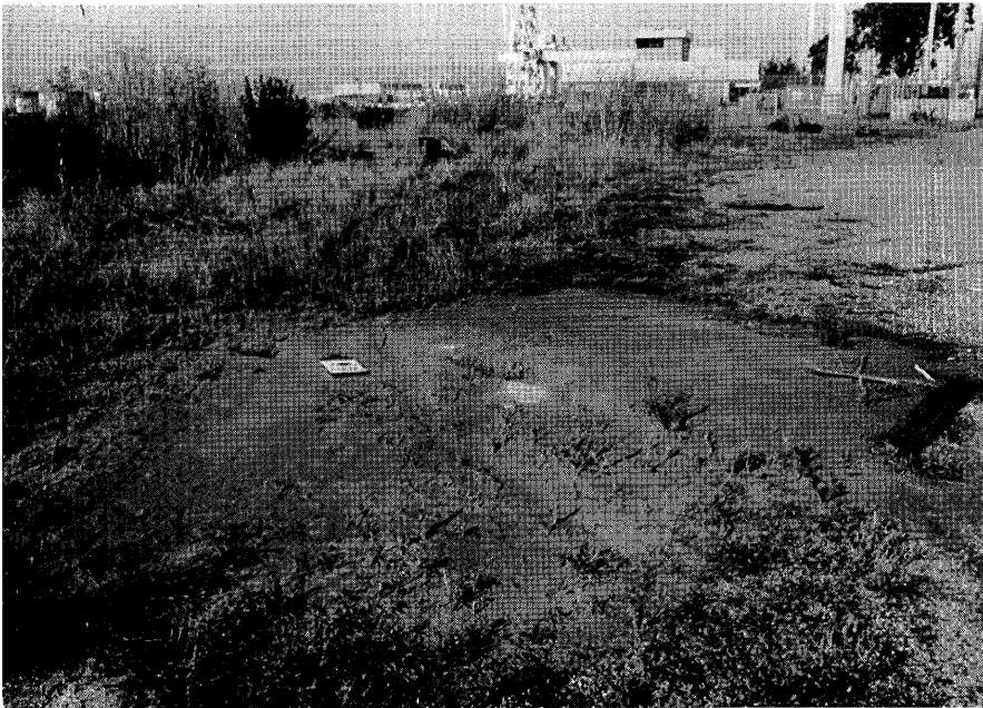
Figure 3.—Sand boils on undeveloped land at end of Harbor Way Road in the Port of Richmond.
