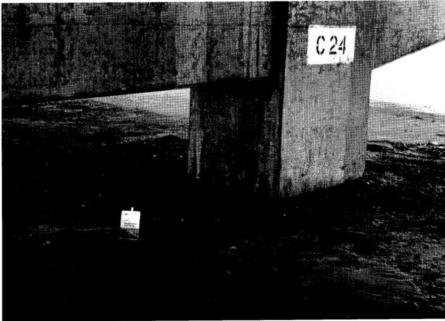
Figure 8.—Sand boils beneath elevated West Grand Avenue distribution structure adjacent to Interstate Highway 80 east of San Francisco Oakland Bay Bridge Toll Plaza.
