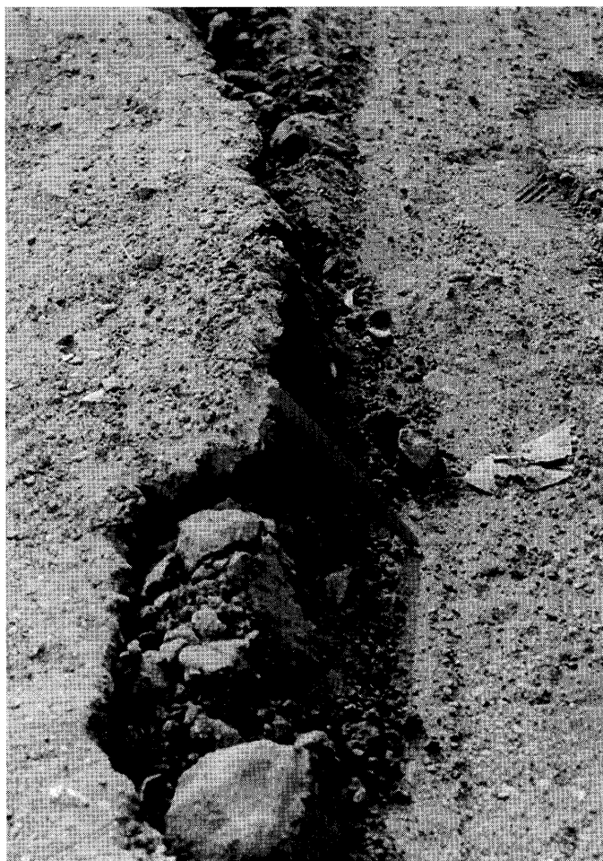
Figure 8.—Typical ground crack observed across from Pier 23 at site 3 (fig. 1). Photograph taken October 19, 1989.
