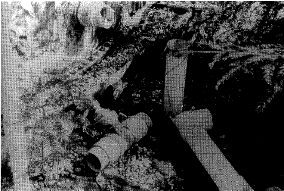
Figure 8.—Tank inlet-outlet piping in the Santa Cruz Mountains damaged because of inadequate flexibility.
