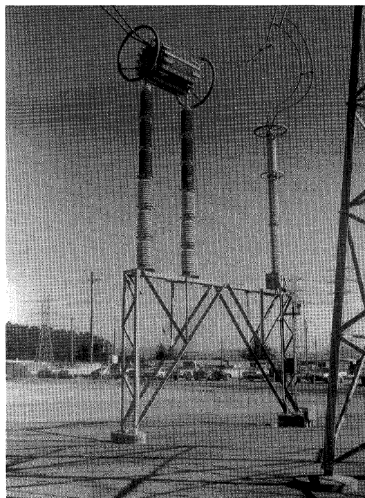
Figure 14.—Line trap and capacitatively coupled voltage transformer on support structure at the Moss Landing Substation (fig. 1).
