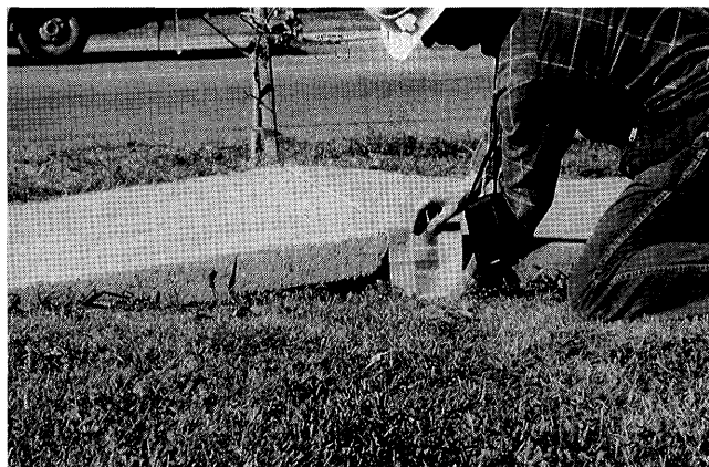
Figure 7.—Buckling of sidewalk in Hollister due to ground settlement.
