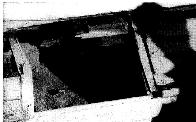
Figure 5.—Typical shear failure of cripple wall in a house in Hollister due to lateral ground motion and insufficient shear connectors.
