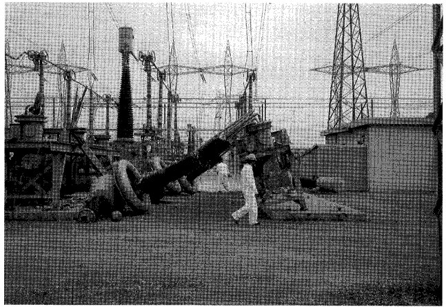
Figure 6.—Overturned 500-kV circuit breaker at the Moss Landing Substation (fig. 1).
