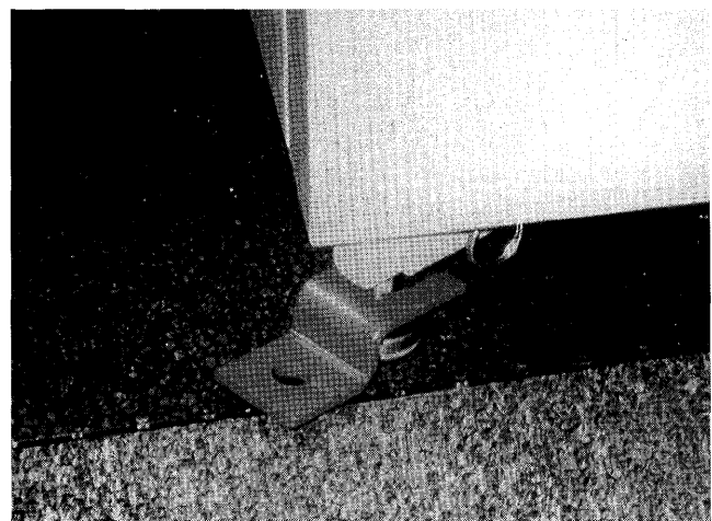
Figure 14.—Typical anchor clip for an electronics cabinet, use to prevent it from overturning.
