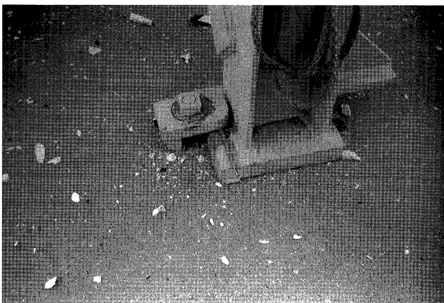
Figure 5.—Friction-clip anchorage of 500-kV circuit breaker at the Moss Landing Substation (fig. 1).
