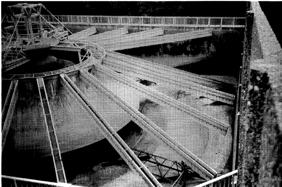
Figure 6.—Damaged water purifier at the Rinconada Water Treatment Plant.
