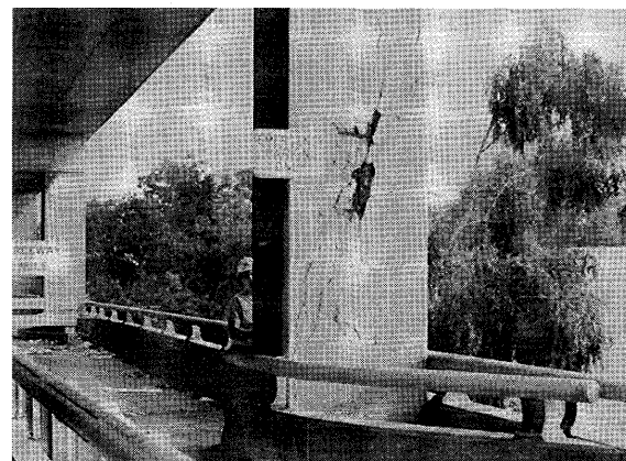
Figure 140.—Damage to Column 2 of Bent 43 at Central Freeway Viaduct (photograph by Mike Van de Pol).
