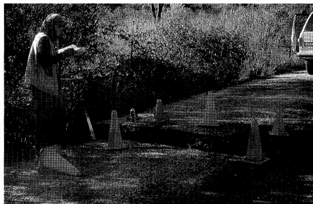
Figure 309.—Damage to Morrill Road from 1989 (Loma Prieta) earthquake.
