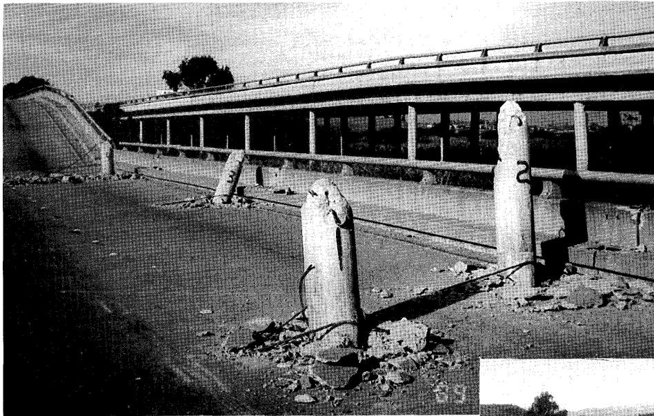
Figure 170.—Piles penetrating deck of left Struve Slough Bridge (view to south).
