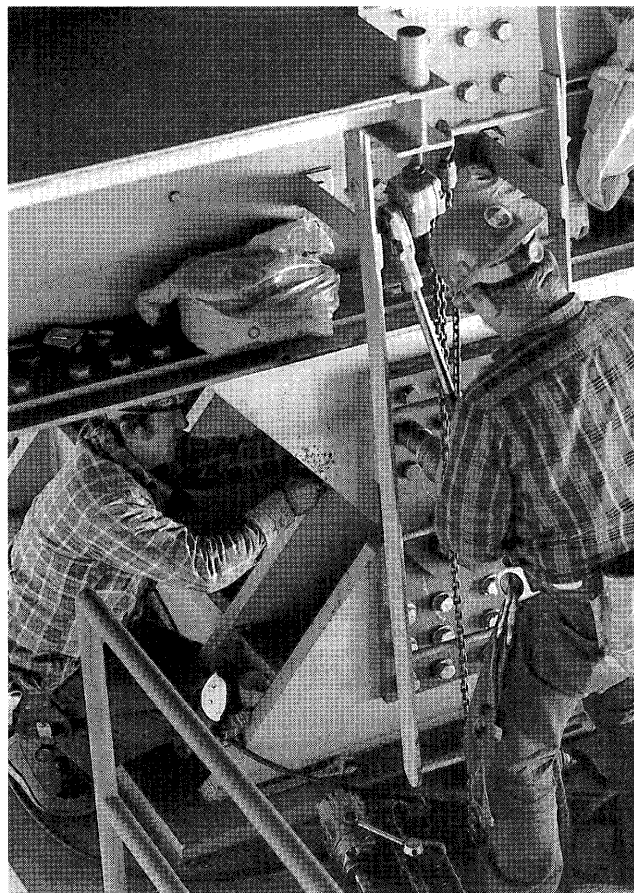
Figure 220.—Repair to damage at Pier 21 of San Mateo-Hayward Bridge.
