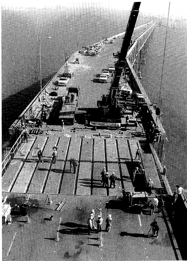
Figure 19.—Installing new, precast deck panels at Pier E9 on East Bay Crossing after the earthquake.
