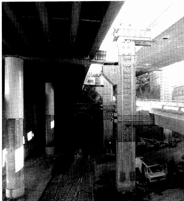
Figure 97.—Damage at Hinge A-44 of China Basin Viaduct (photograph by Mike Van de Pol).
