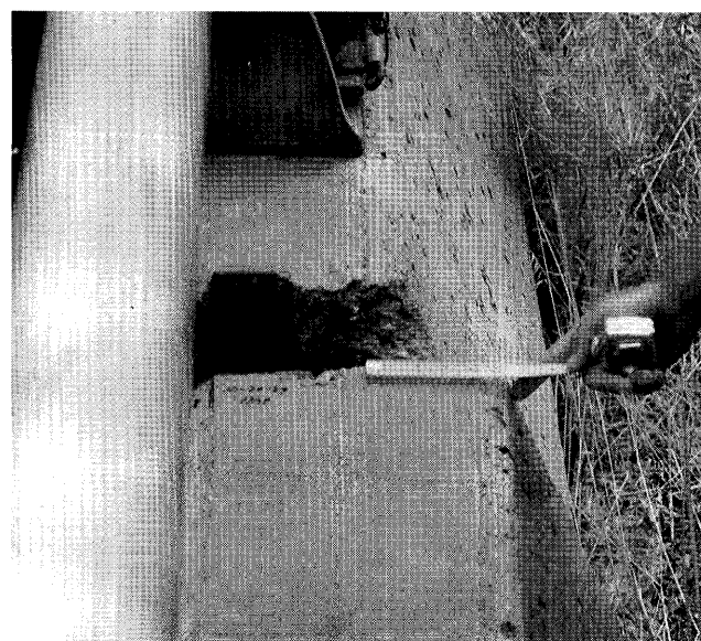
Figure 232.—Horizontal offset of west abutment at Mora Drive Overcrossing (courtesy of Earthquake Engineering Research Institute).
