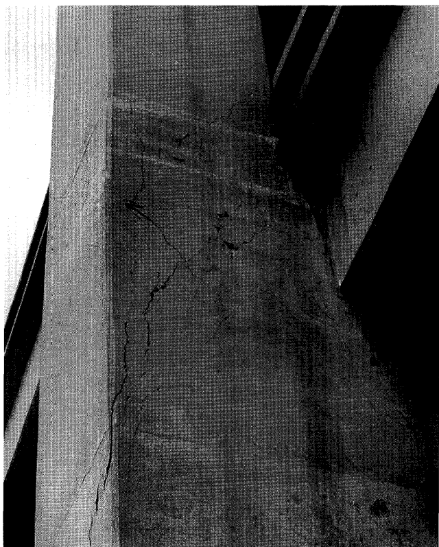
Figure 119.—Column damage to west side of Bent 79 at Embarcadero Viaduct.
