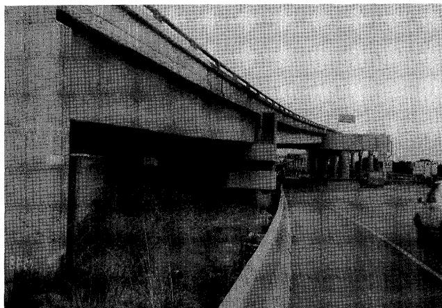
Figure 145.—Completed retrofit for Alemany Interchange.
