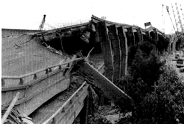
Figure 27.—Pin connection failure at Cypress Viaduct.
