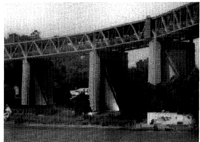
Figure 20.—Proposed retrofit of encasing steel towers in concrete for East Bay Crossing (currently (1997) superseded by plans to replace this structure).
