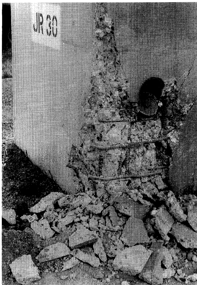
Figure 55.—Spalling at southeast face of Bent 30 on JR line of Port of Oakland Overcrossing (photograph by Li Hong Sheng).
