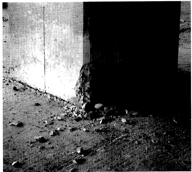
Figure 71.—Spall at column base for Bent 35 of Fifth Avenue Overhead (courtesy of Earthquake Engineering Research Institute).
