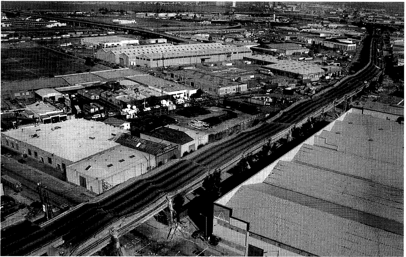
Figure 30.—Collapse of Cypress Viaduct between Bent 62 and Bent 113.
