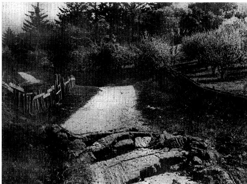
Figure 310.—Similar damage to Morrill Road from 1906 earthquake.
