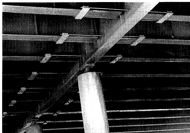
Figure 243.—Existing bearings (before removal) during retrofit of Sierra Point Overhead.
