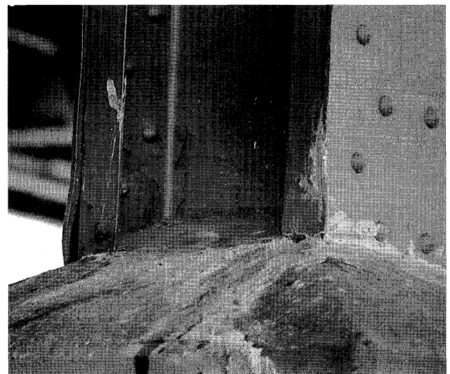
Figure 76.—Steel column damage at Fifth Avenue Overhead (courtesy of Abolhassan Astaneh-Asl).
