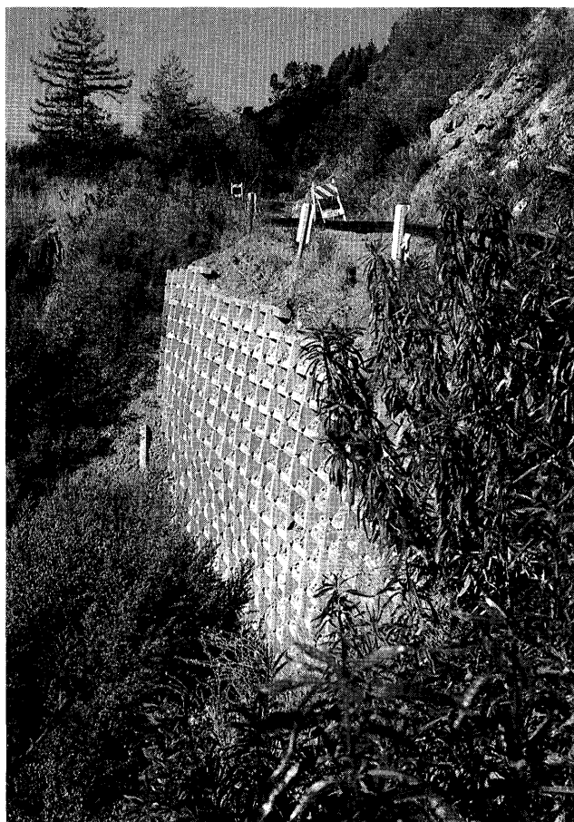
Figure 324.—Crib wall (courtesy of Earthquake Engineering Research Institute).
