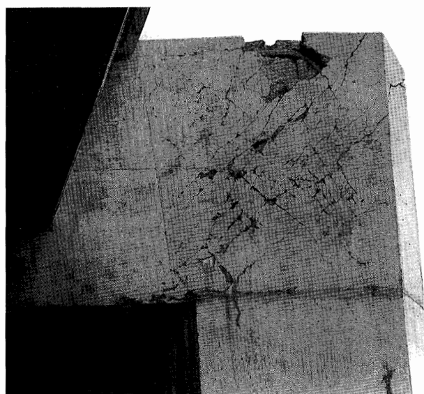
Figure 4.—Damage to outrigger knee-joint on Route 980 Southbound Connector.
