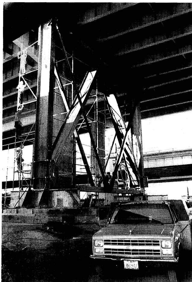
Figure 64.—Emergency Repairs to the Distribution Structure.
