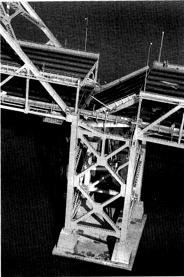
Figure 12.—Fallen decks at Pier E9 of the East Bay Crossing.
