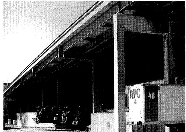
Figure 75.—Location of steel columns at Fifth Avenue Overhead (courtesy of Abolhassan Astaneh-Asl).
