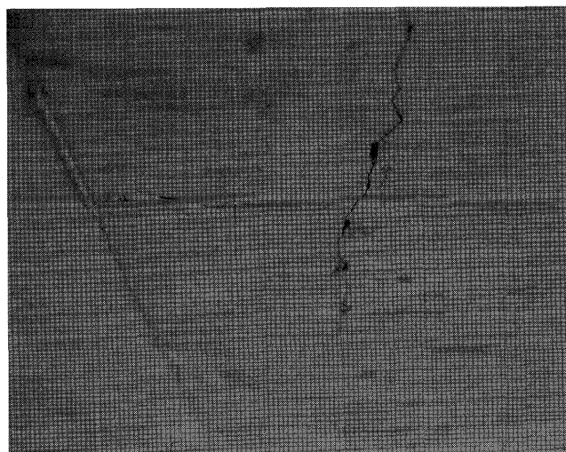
Figure 160.—Soffit cracks on Northeast Connector of Route 92/101 Interchange.
