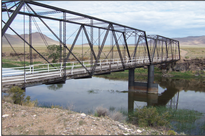
Figure 4. Photograph of the Costilla Crossing Bridge over the Rio Grande. The bridge is a single lane, two-span Thatcher through-truss bridge constructed in 1892. It was posted to the National Register of Historic Places in 1985. The bridge is 11.5 km south of Colorado Hwy 142 bridge over the Rio Grande and accommodates local traffic in the southern San Luis Valley. Oligocene intrusive rocks (Tiq) of South Piñon Hills (left) and mesa-capping basaltic lava flows (Th) overlying andesite lava flows (Tcl) of Piñon Hills (right) are visible in background. The bridge rests on a single Servilleta Basalt (Tsb) lava flow likely erupted from vent(s) to the south. The bridge was restored in 2006. Photo by Ren A. Thompson, 2005.
