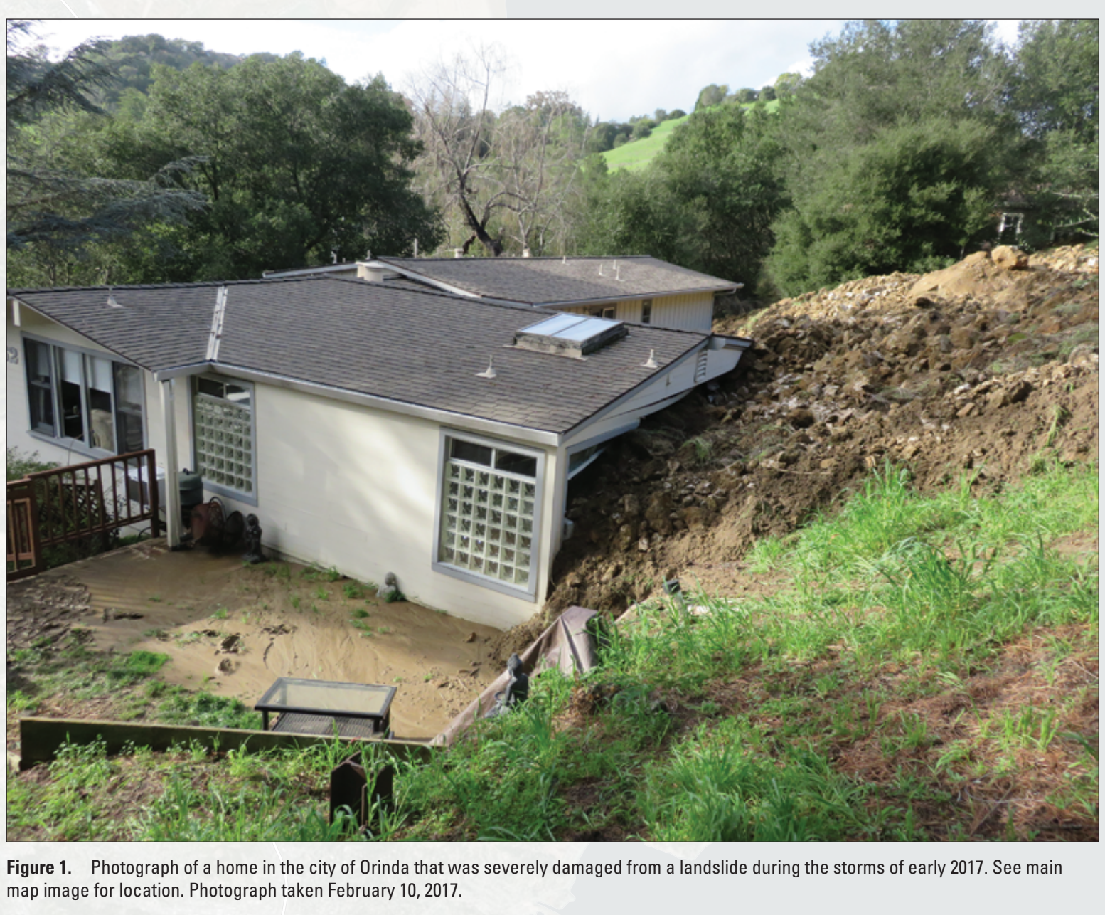
Figure 1. Photograph of a home in the city of Orinda that was severely damaged from a landslide during the storms of early 2017. See main map image for location. Photograph taken February 10, 2017.
