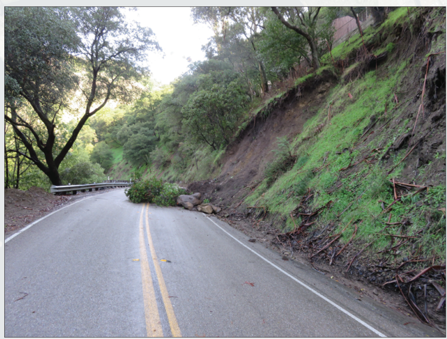
Figure 4. Photograph showing a road partly blocked by a shallow landslide along a steep cut slope, one of many blockages that occurred during the storms of early 2017. Some roads remained blocked for several months as crews worked to stabilize saturated hillslopes. See main map image for location. Photograph taken January 23, 2017.
