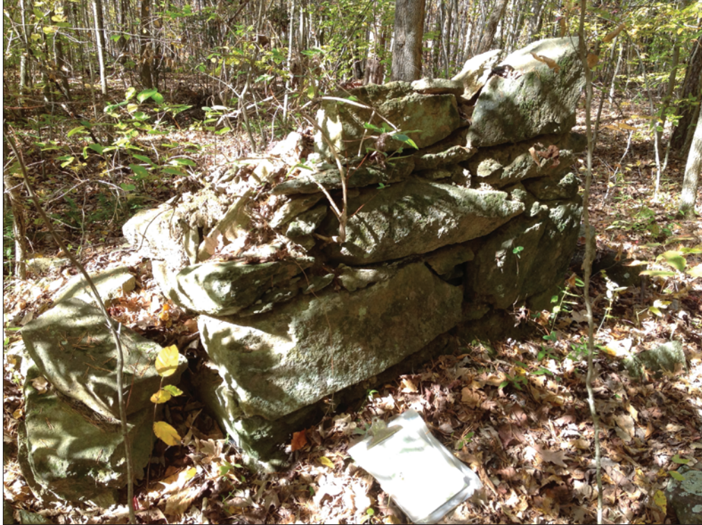
Figure 21. Photograph of rough-hewn and uncut field stones of altered ultramafic rock (soapstone; map unit Ocum) that were used as foundation blocks in the Buckner 7.5-minute quadrangle (photograph locality 27 on the map). The map board (approximately 23 centimeters wide) is shown for scale. Photograph by Mark Carter, U.S. Geological Survey.
