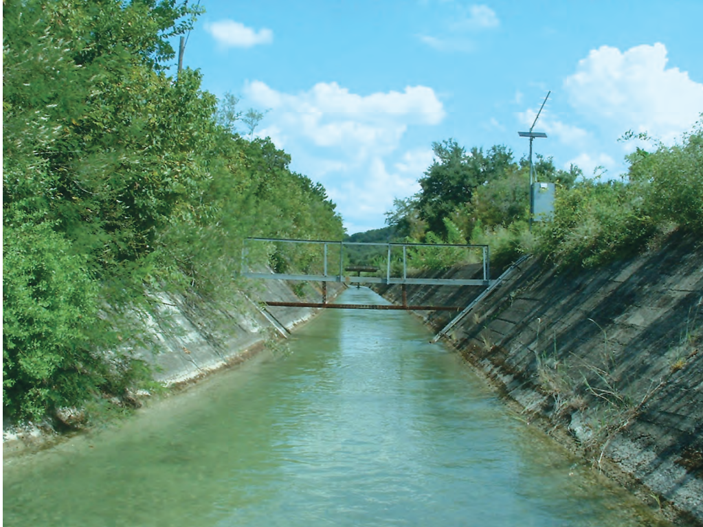
Figure 5. Medina Irrigation Canal near Riomedina, Texas, August 2004.
