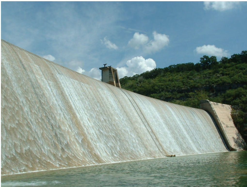
Figure 6. Diversion Dam near Riomedina, Texas, August 2004.
