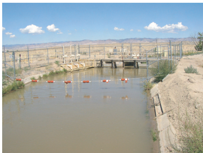
Figure 7. Government Highline Canal at Camp 7 near Highline Lake, Grand Junction, Colorado, August 23, 2003, when the measured turbidity was 66 nephelometric turbidity units.
