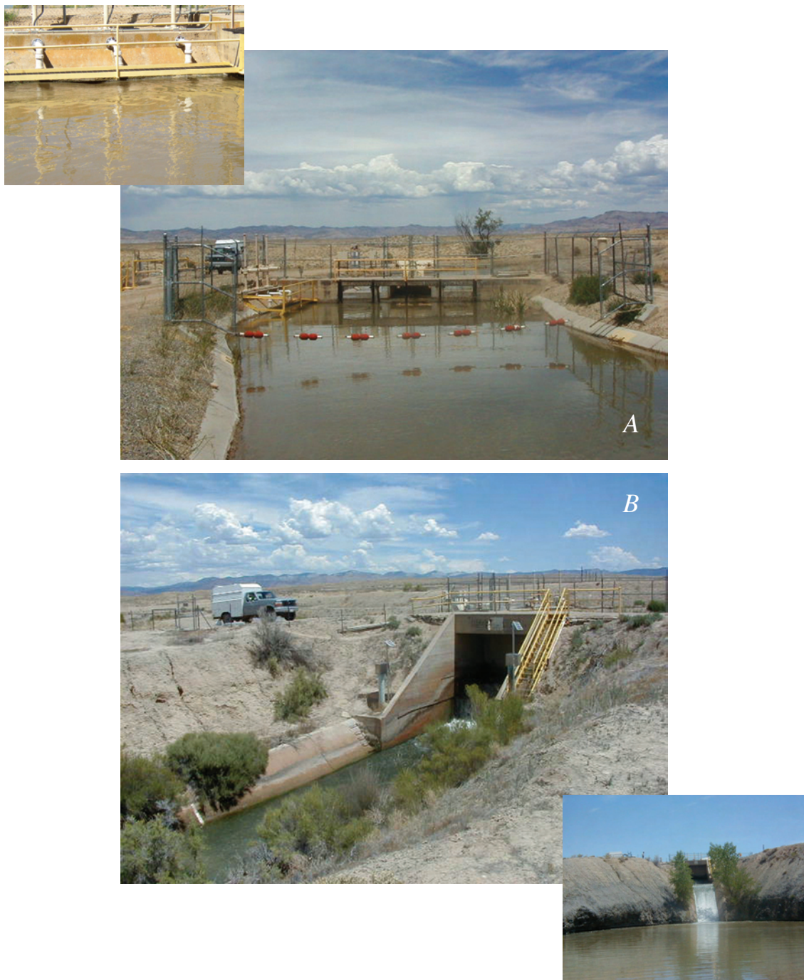
Figure 3. (A) Camp 7 sampling location just upstream from check structure on the Government Highline Canal with inset of siphon works to spillway, and (B) view of Camp 7 spillway with inset of inflow to Highline Lake.
