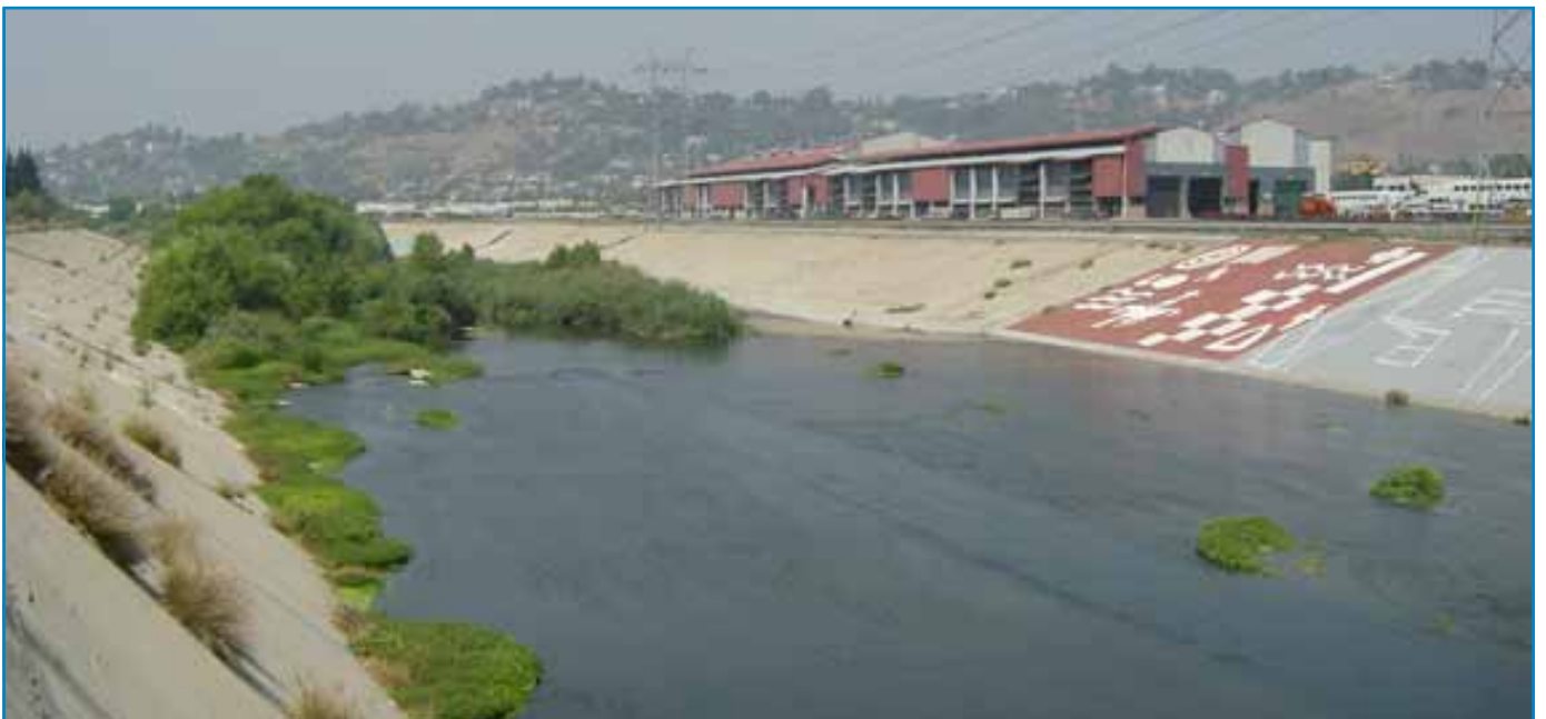
Upstream view near an unlined section of the Los Angeles River. (photograph by Dale Cox, U.S. Geological Survey)
