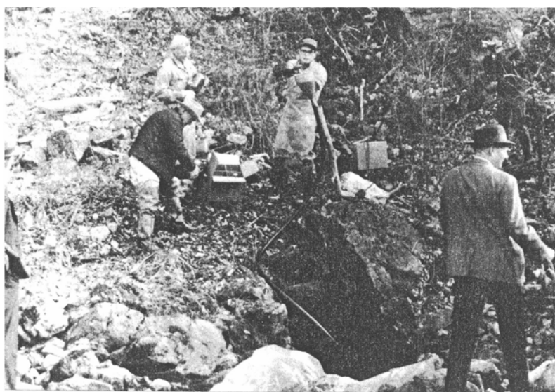
Figure 4. Injecting dye in 1968 into the swallow hole in the Pahasapa Limestone along Boxelder Creek near Custer Gap (From Rahn and Gries, 1973).
