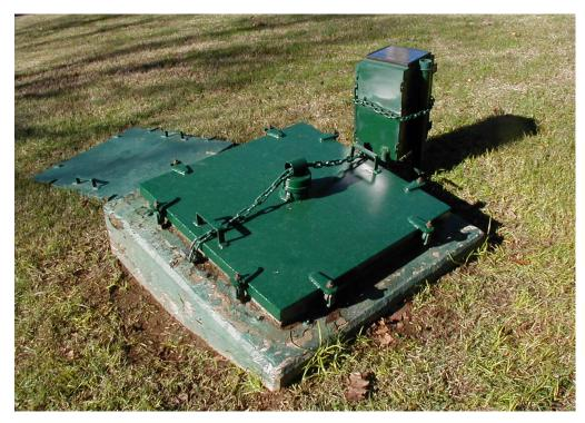
Figure 5. Collection box 2 with fabricated lid to provide access for dye trace monitoring, Hot Springs National Park, Arkansas.
