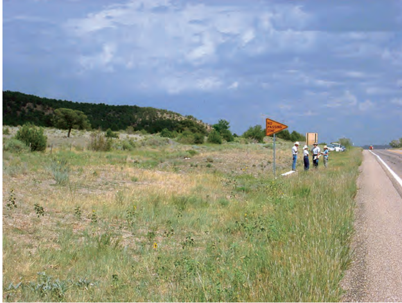
Figure A156. Site of culvert measurement, Cimarron Creek Tributary near Cimarron, New Mexico, August 5, 2003.
