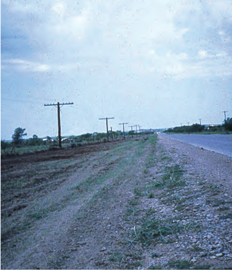
Figure A16. Upstream side of State Highway 6 overflow near right bank looking toward left bank with rod held near fence at the high-water mark in the approach section, North Fork Hubbard Creek near Albany, Texas, August 15, 1978.
