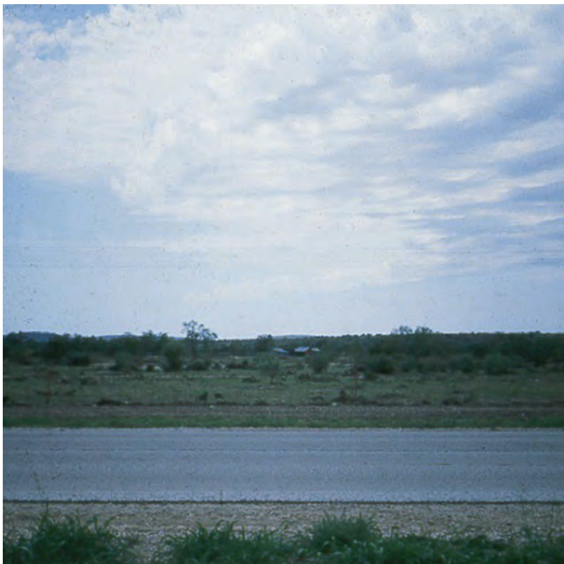
Figure A29. View from 25 feet downstream of State Highway 6 near left end of overflow looking upstream at approach section. Main channel in background is North Fork Hubbard Creek near Albany, Texas, August 15, 1978.
