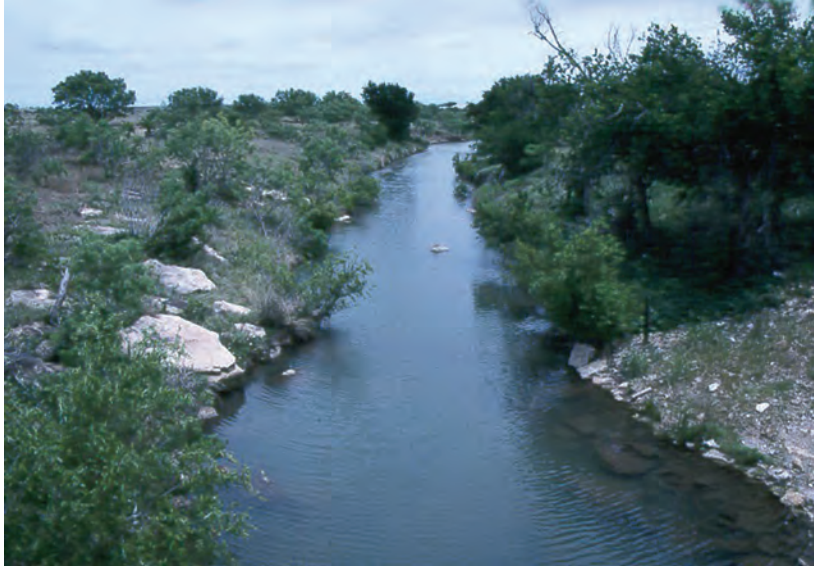
Figure A38. View looking downstream of State Highway 6 bridge, North Fork Hubbard Creek near Albany, Texas, May 12, 2003.
