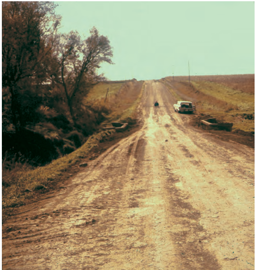
Figure A218. View of left bank high-water mark at bridge crossing, Stratton Creek near Washta, Iowa, August 1961. Flow is from left to right.
