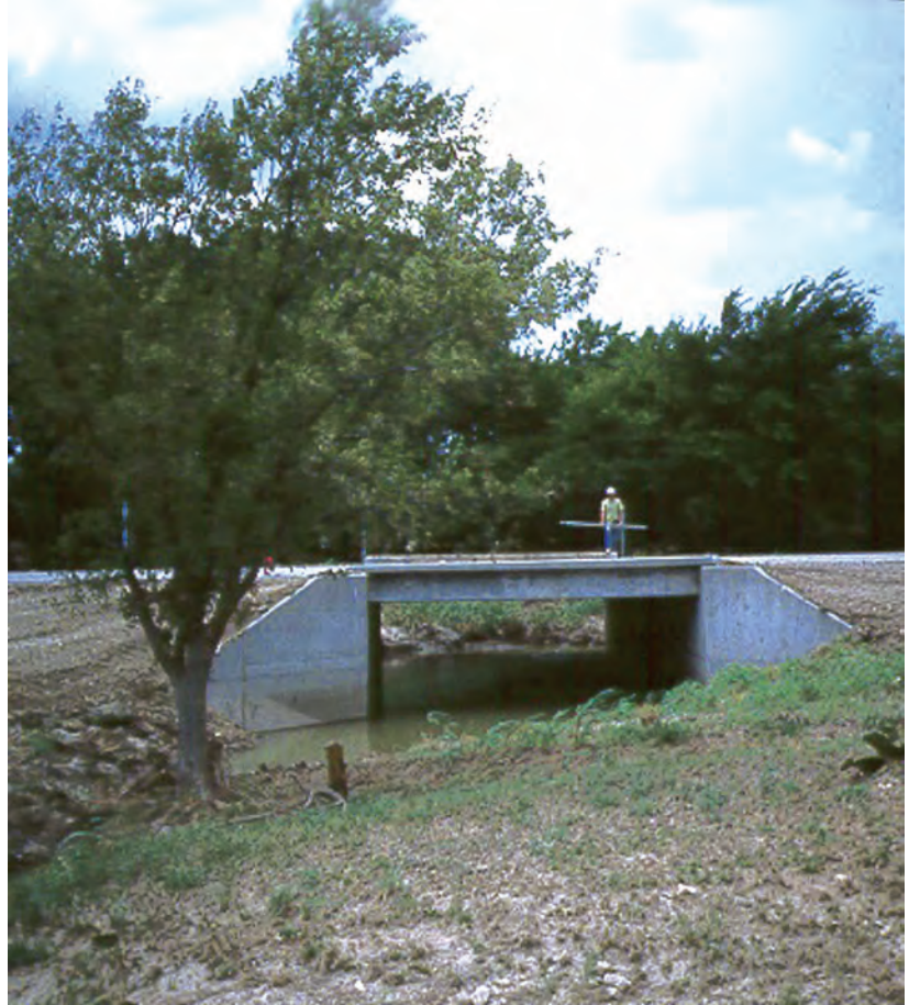
Figure A24. View from about 100 feet downstream of culvert located to right of gaging station looking upstream at culvert and approach section with rod held on upstream side of culvert near high-water mark in approach section, North Fork Hubbard Creek near Albany, Texas, August 15, 1978.
