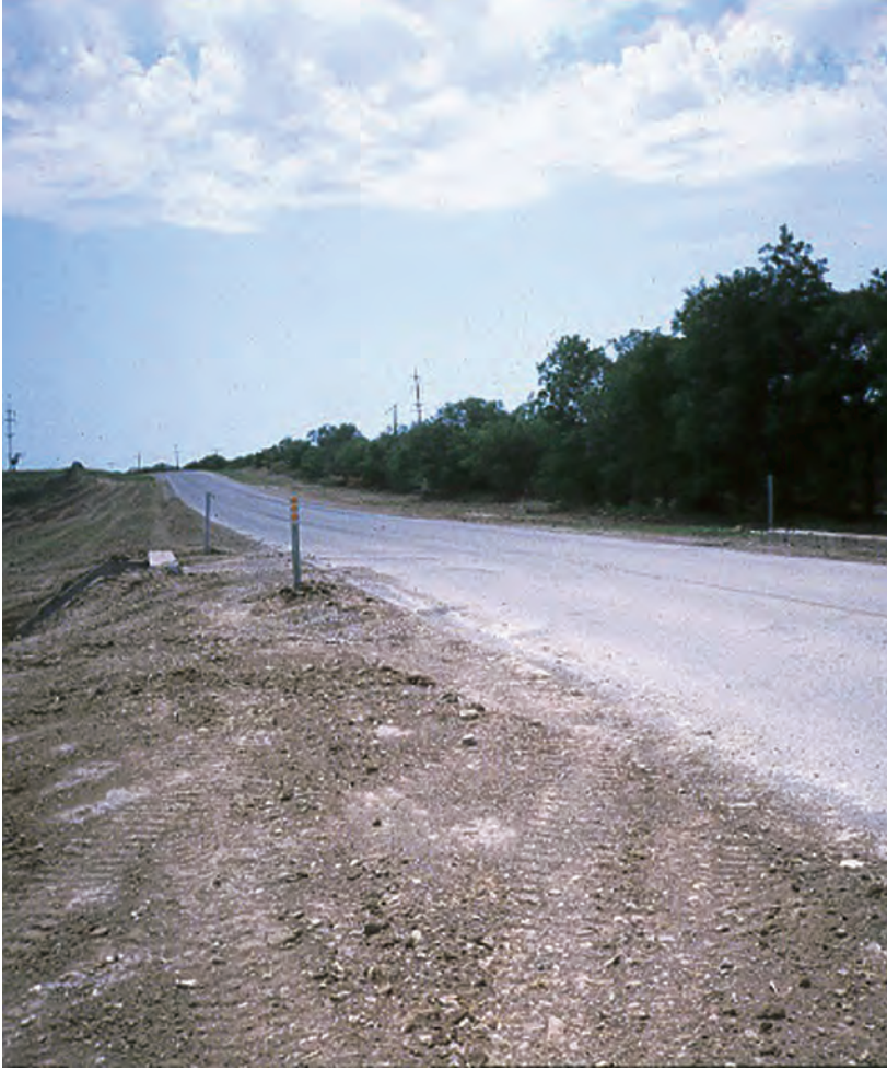
Figure A26. View about 100 feet to left of culvert on downstream shoulder of State Highway 6 looking across culvert at right bank and approach section. Rod held at high-water mark in approach, North Fork Hubbard Creek near Albany, Texas, August 15, 1978.
