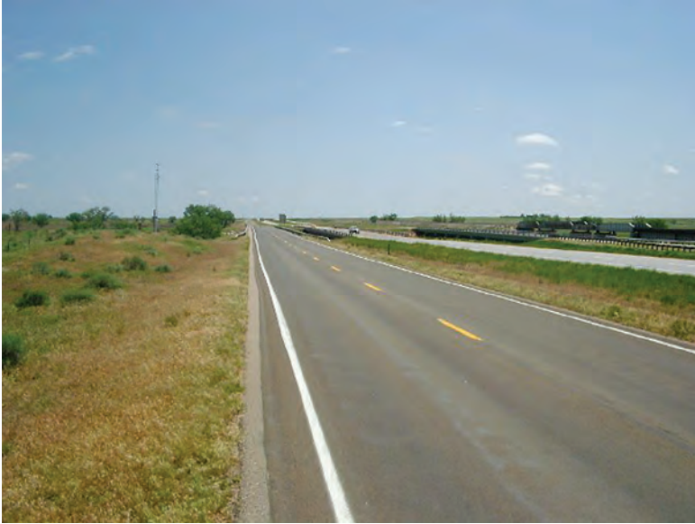
Figure A92. View looking north toward railroad wash-out, Bijou Creek near Wiggins, Colorado, June 3, 2003.
