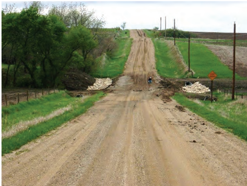
Figure A226. View looking from right to left bank along road crossing, Stratton Creek near Washta, Iowa, May 5, 2003.
