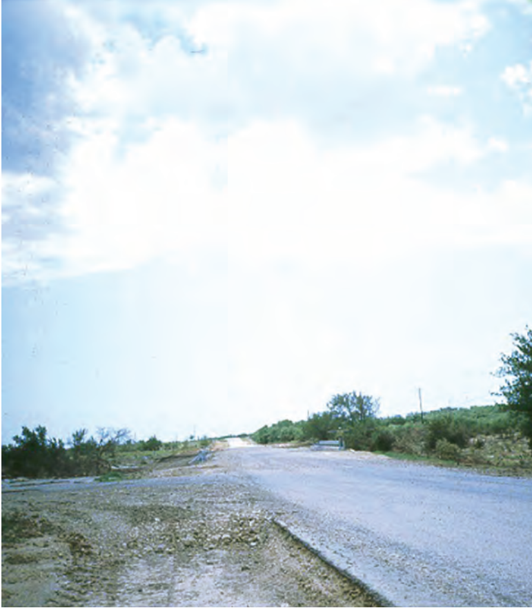
Figure A20. View from about 200 feet to left and 25 feet downstream of gaging station at bridge looking right and across at approach section and right bank. Rod held near high-water mark in approach section, North Fork Hubbard Creek near Albany, Texas, August 15, 1978.
