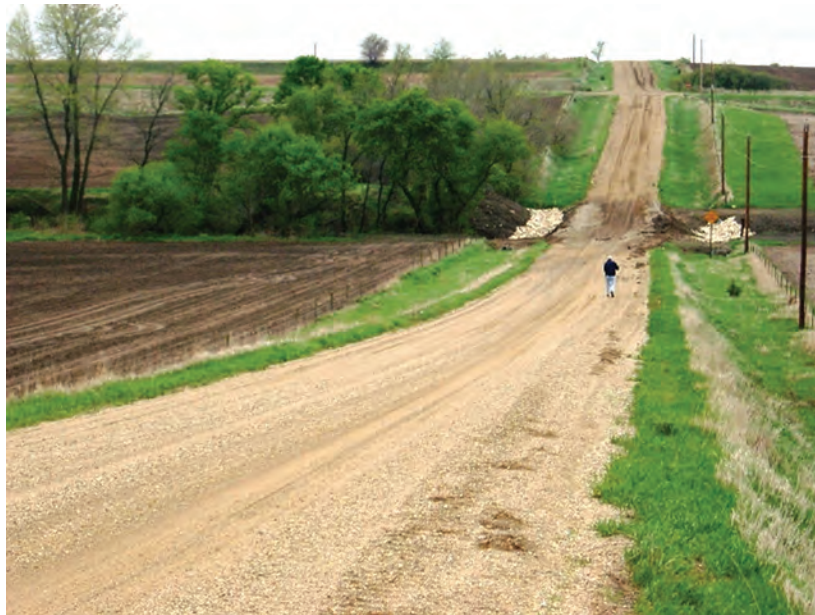
Figure A230. View looking from right to left bank at culvert crossing, Stratton Creek near Washta, Iowa, May 5, 2003. Flow is from left to right.
