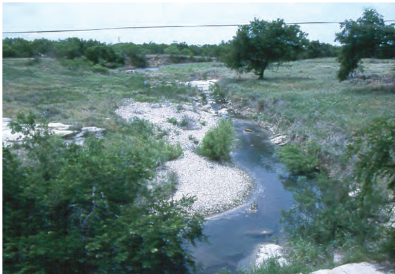
Figure A37. View looking upstream of State Highway 6 bridge, North Fork Hubbard Creek near Albany, Texas, May 12, 2003.
