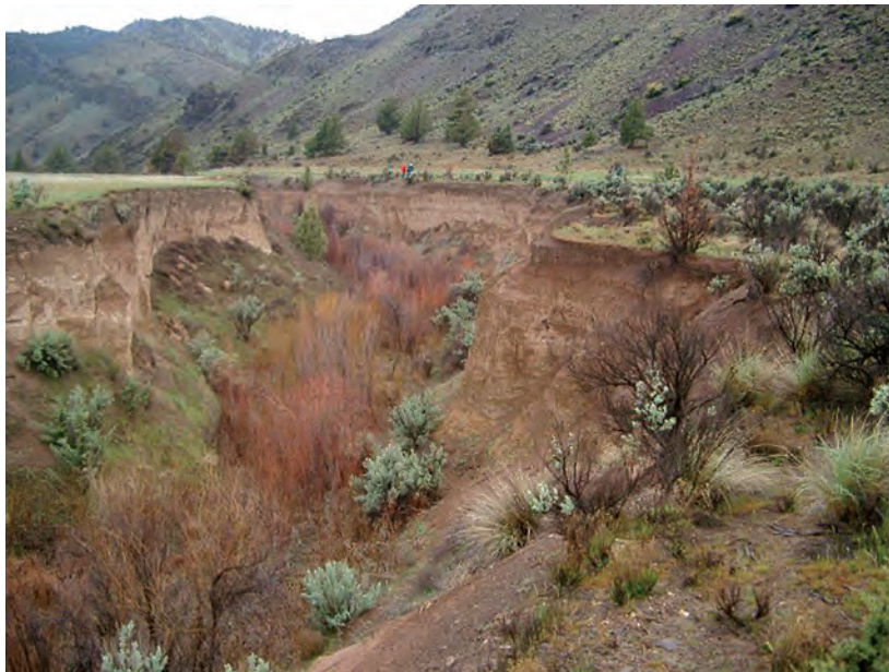
Figure A170. View looking downstream into main canyon toward slope-area reach, Meyers Canyon near Mitchell, Oregon, April 21, 2003.
