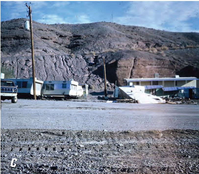
Figure A143. Damage to trailers (a), Eldorado Canyon at Nelson Landing, Nevada, September 1974.—Continued.
