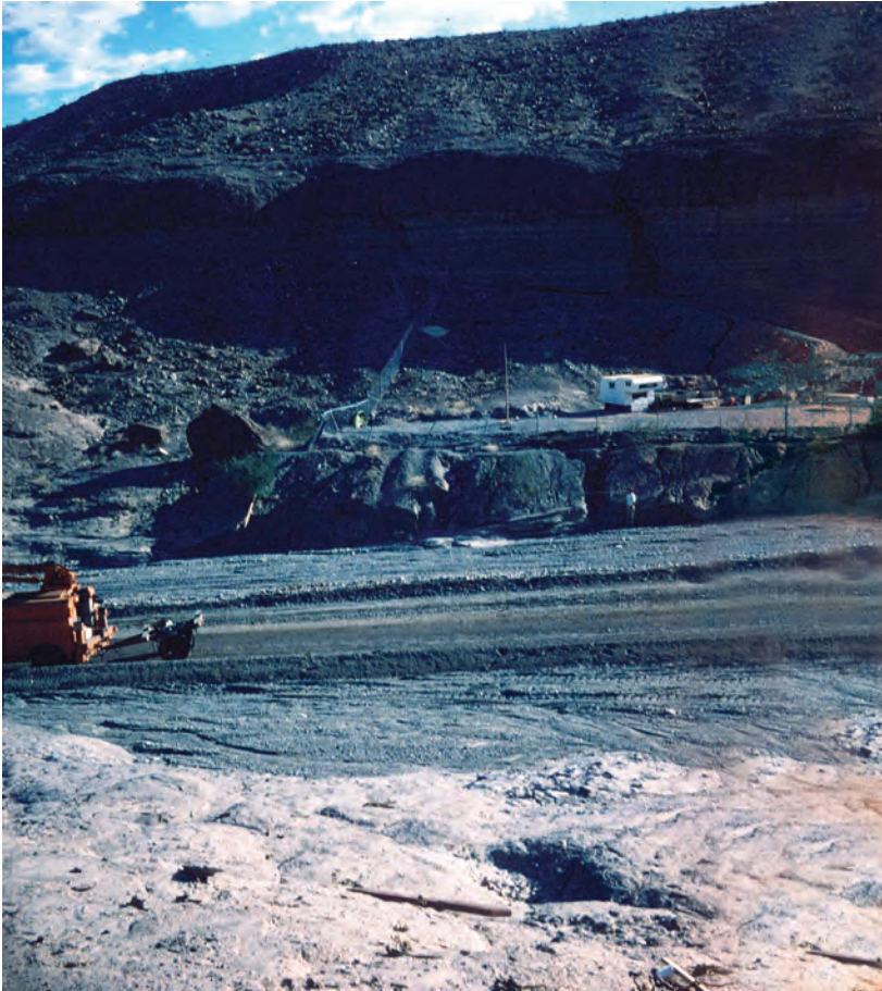
Figure A122. View of trailers from left bank to right bank, Eldorado Canyon at Nelson Landing, Nevada, September 1974.
