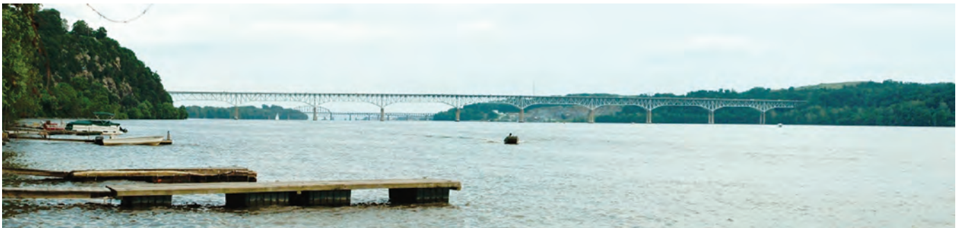
Figure A246. View upstream of Interstate Highway I-95 bridge across Susquehanna River where current-meter measurement was made of June 24, 1972 flood, Susquehanna River at Conowingo, Maryland.
