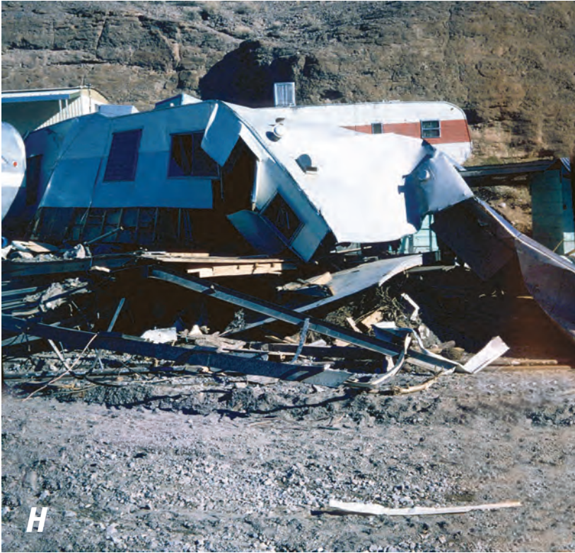
Figure A143. Damage to trailers (a), Eldorado Canyon at Nelson Landing, Nevada, September 1974.—Continued.
