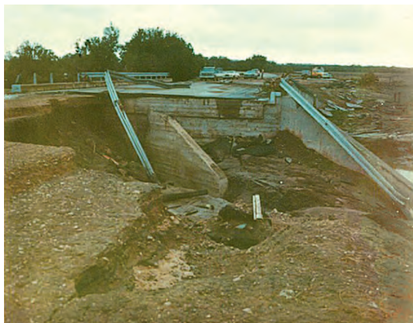
Figure A7. View from right end of bridge looking across bridge, North Fork Hubbard Creek near Albany, Texas, August 5, 1978. Flood of August 4, 1978, was about 2 feet over handrail.
