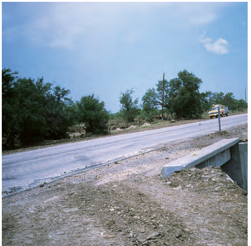
Figure A27. View from 50 feet to right of culvert on downstream shoulder looking across culvert with rod held at high-water mark in approach section, North Fork Hubbard Creek near Albany, Texas, August 15, 1978.
