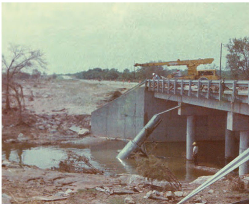
Figure A14. View of bridge and channel downstream from left bank, shelter and well being lifted out of stream, North Fork Hubbard Creek near Albany, Texas, August 10, 1978.
