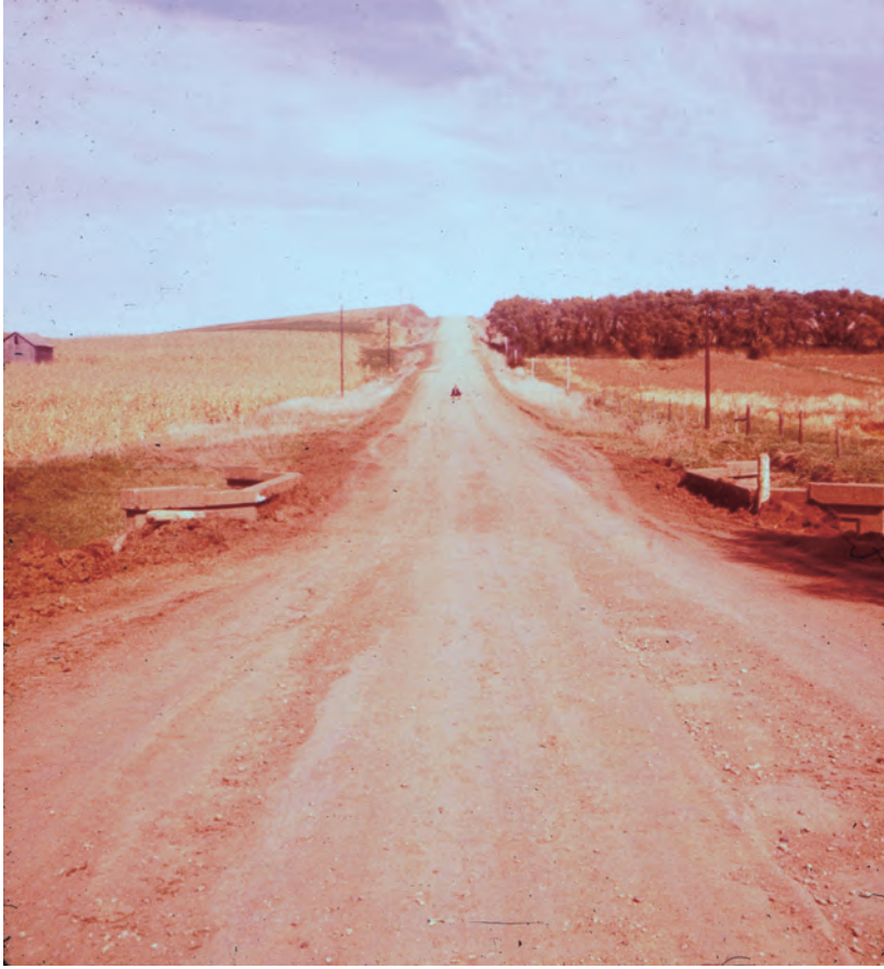
Figure A213. View of right-bank high-water mark at bridge crossing, Stratton Creek near Washta, Iowa, August 1961. Flow is from right to left.
