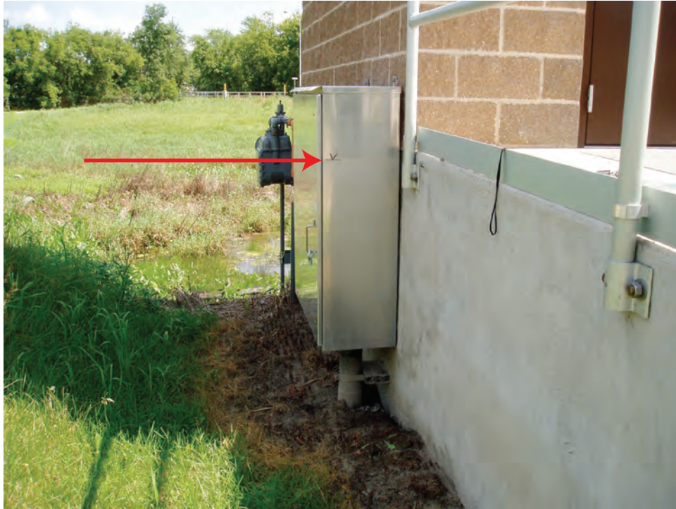
A. Reedsburg high-water mark 2, mudline on electrical box of sewage pump station, corroborated with city of Reedsburg mark surveyed in June during high water.
