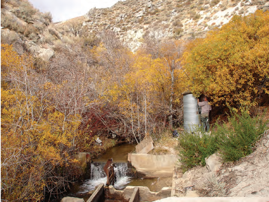
Figure 15. View looking upstream at site 2, Clear Creek near Carson City (10310500), Douglas County, Nevada. Photograph taken by Ralph Seiler, U.S. Geological Survey, November 8, 2006.
