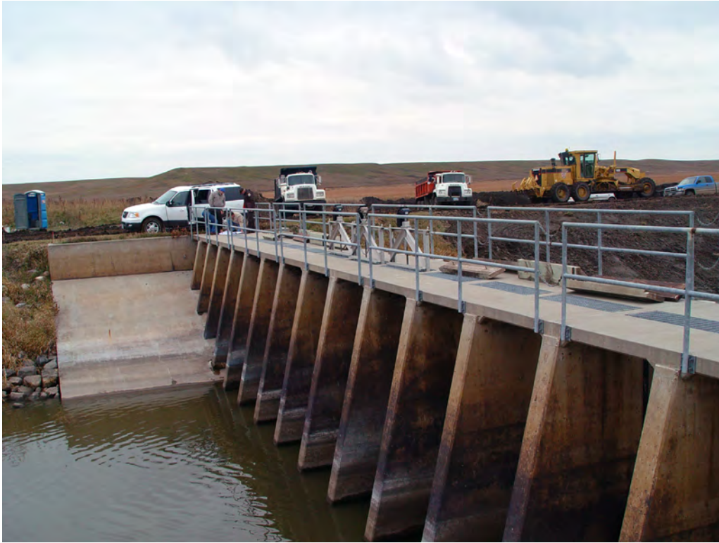
Figure 4. Depuy control structure on Jim Lake drawdown channel near south end of Arrowwood National Wildlife Refuge, October 2006.
