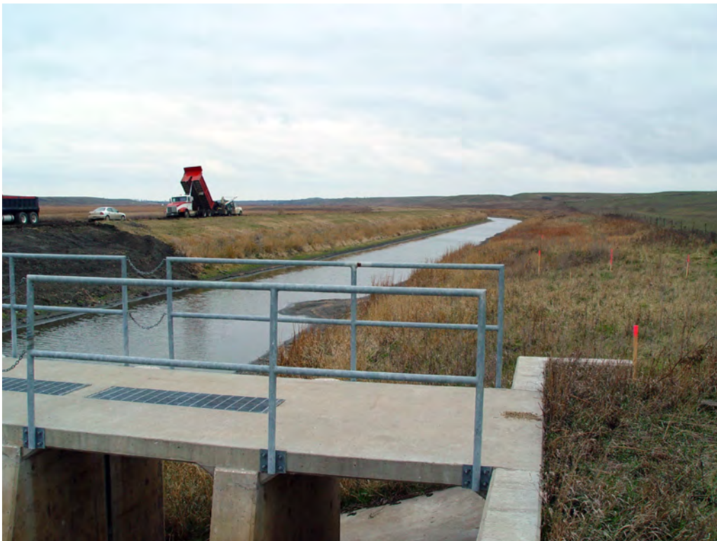
Figure 3. Jim Lake drawdown channel and DePuy control structure near south end of Arrowwood National Wildlife Refuge, October 2006.
