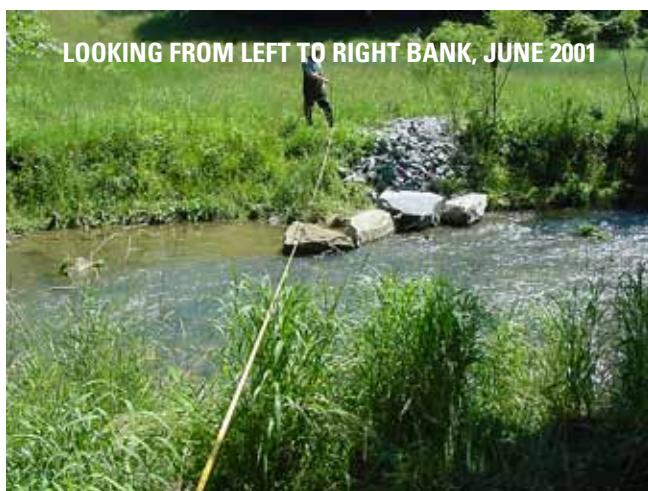
Figure 4–2. Views of the upstream rock deflector and cross section during the initial survey in June 2001 and last survey in September 2006.
