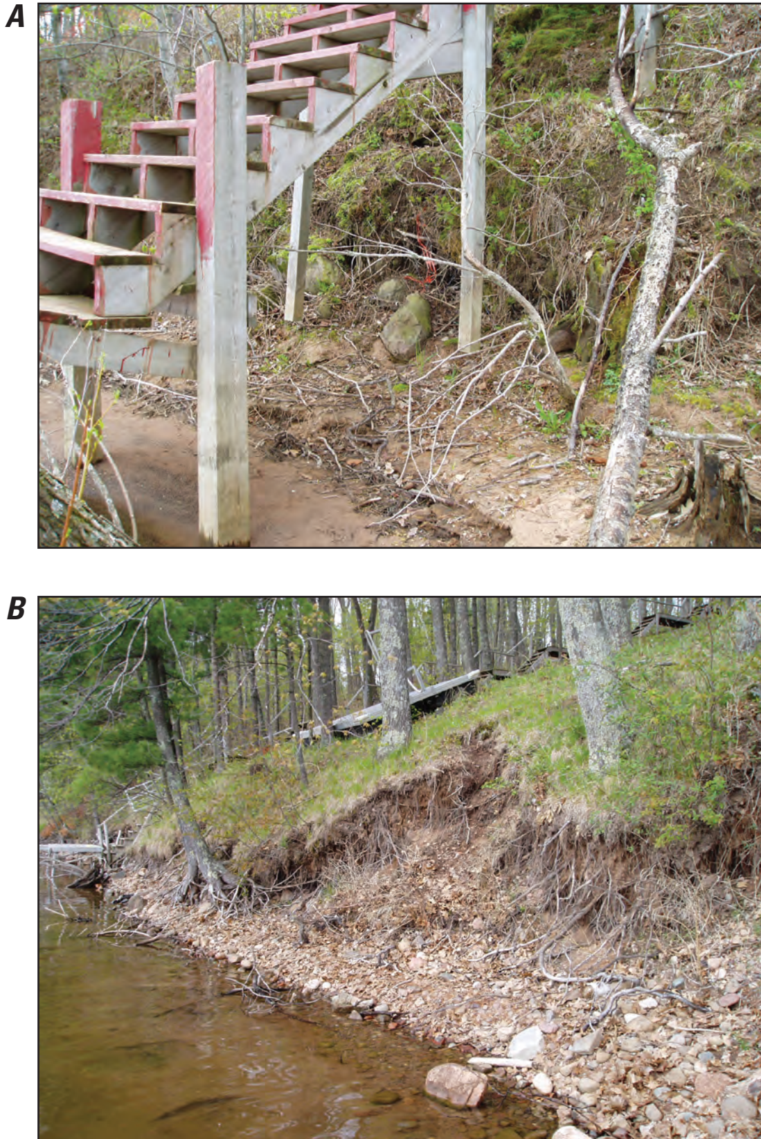
Figure 18. Erosion at two locations on Silver Lake, Barron County, Wis. A , Site 3 near county park, with erosion around the support beams of the steps down to the water. Notice that the middle support beams are hanging in the air. B , Site 21, demonstrating examples of erosion on the east side of the lake. Site locations shown in figure 3.
