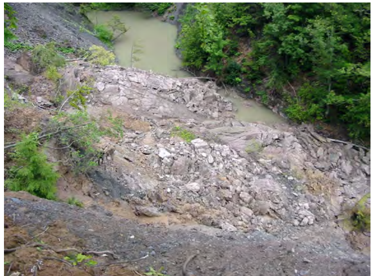
Slope failure which blocked Rattlesnake Gulf, Spring 2006.
