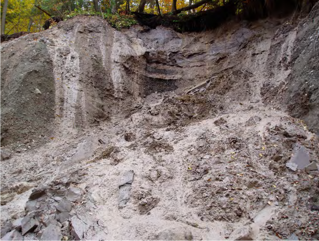
Failure of upper scarp of sand and gravel, revealing laminated and tilted silt and clay unit with overlying till at Rainbow Creek landslide.
