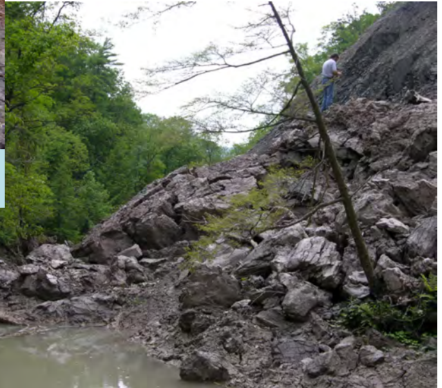
Toe of slope failure which blocked Rattlesnake Gulf, Spring 2006
