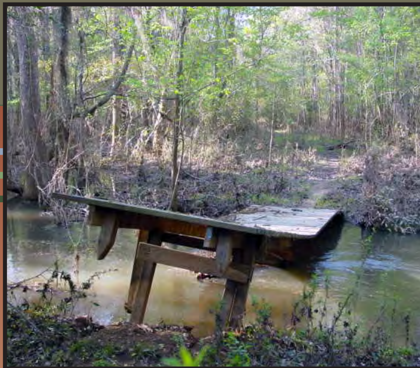
Figure 14. Photograph of damaged trail bridge across a narrow drain in Congaree National Park following high floods in spring of 2003.
