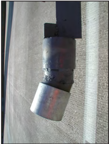
Three-inch galvanized steel pipe angled to clear footer and seal course, with enclosed transducer head flush with pipe. Note 3-inch angle welded to casing.
