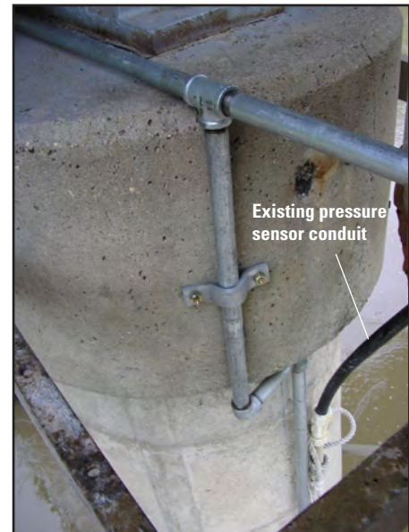
Installation of pipe junction to accommodate the downstream and the upstream river channel-bed monitor cables. Note the galvanized steel pipe that is parallel to the existing conduit for the pressure transducer on the downstream column.
