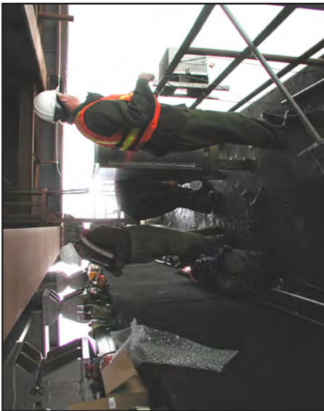
Wiring of river channel-bed monitors and non-contact water surface sensor to a shelter housing the NEMA 0183 to SDI-12 data conversion devices and data collection platform.
