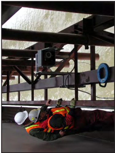
Installation of non-contact water surface sensor clamped to girders underneath bridge.
