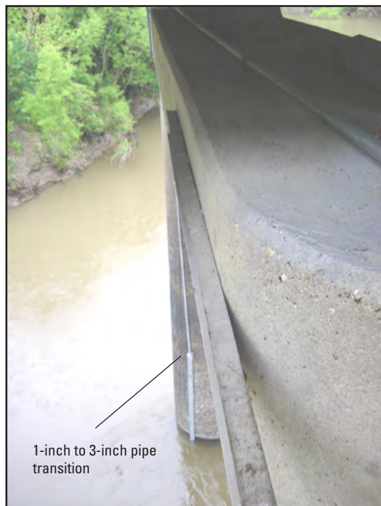
Installation of galvanized steel pipe along the top of the cap and continuing along the downstream side of the upstream conical column. Note the 1-inch to 3-inch pipe transition to accommodate the transducer head below the water surface.
