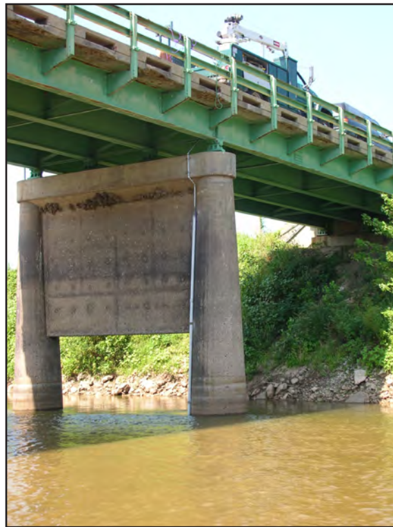
Installation of 1-inch to 3-inch galvanized steel pipe encasing the transducer head and shielded cable on the downstream side of the upstream conical column of pier 4 and between girders.
