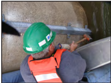
Installation of shielded cable in 1-inch steel pipe under 3-inch steel angle with expandable anchor bolts.
