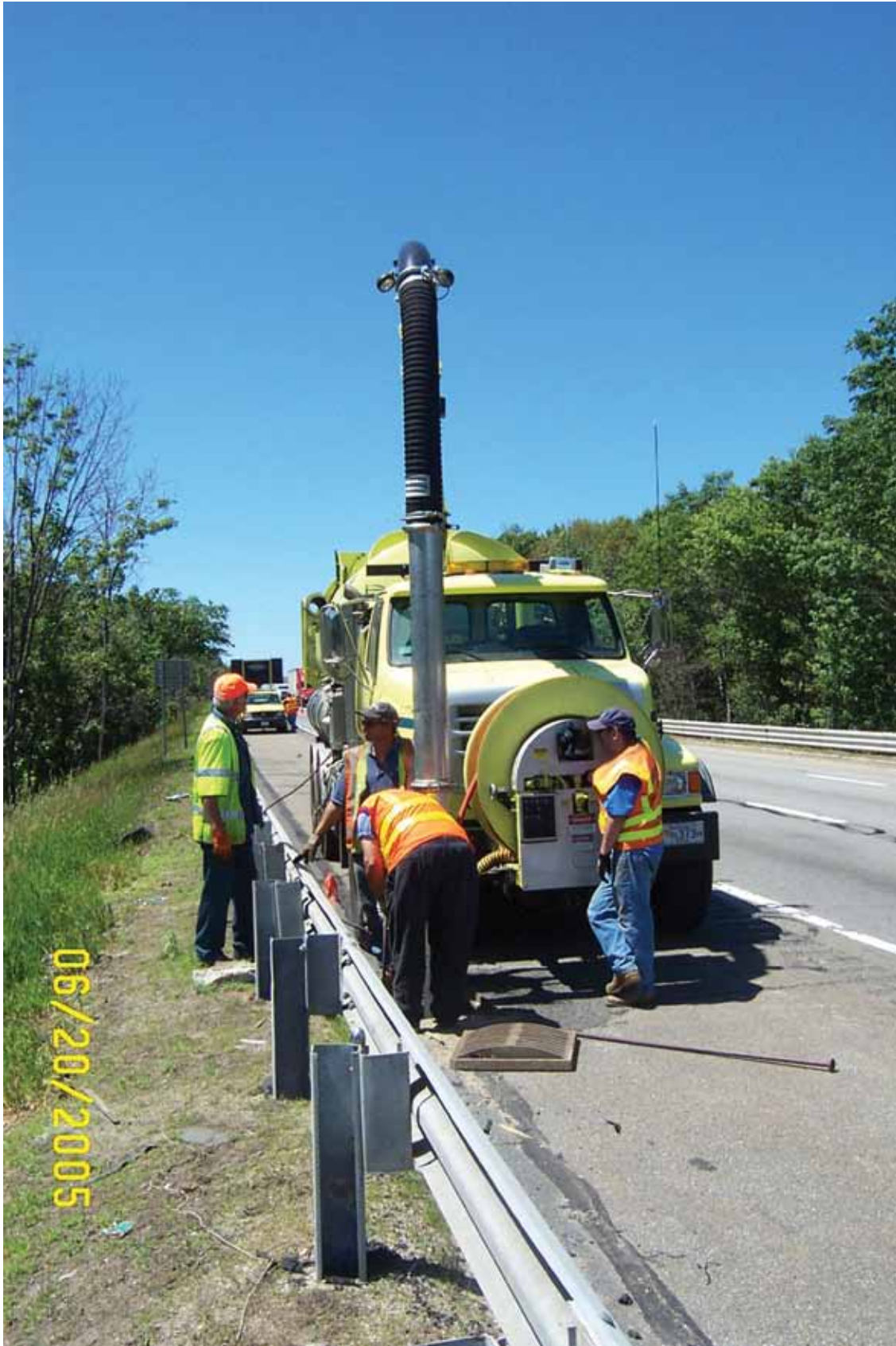
Figure 3. A catch basin at the highway-monitoring station on Interstate 495 being cleaned by Massachusetts Department of Transportation personnel with a vacuum truck prior to the start of monitoring.
