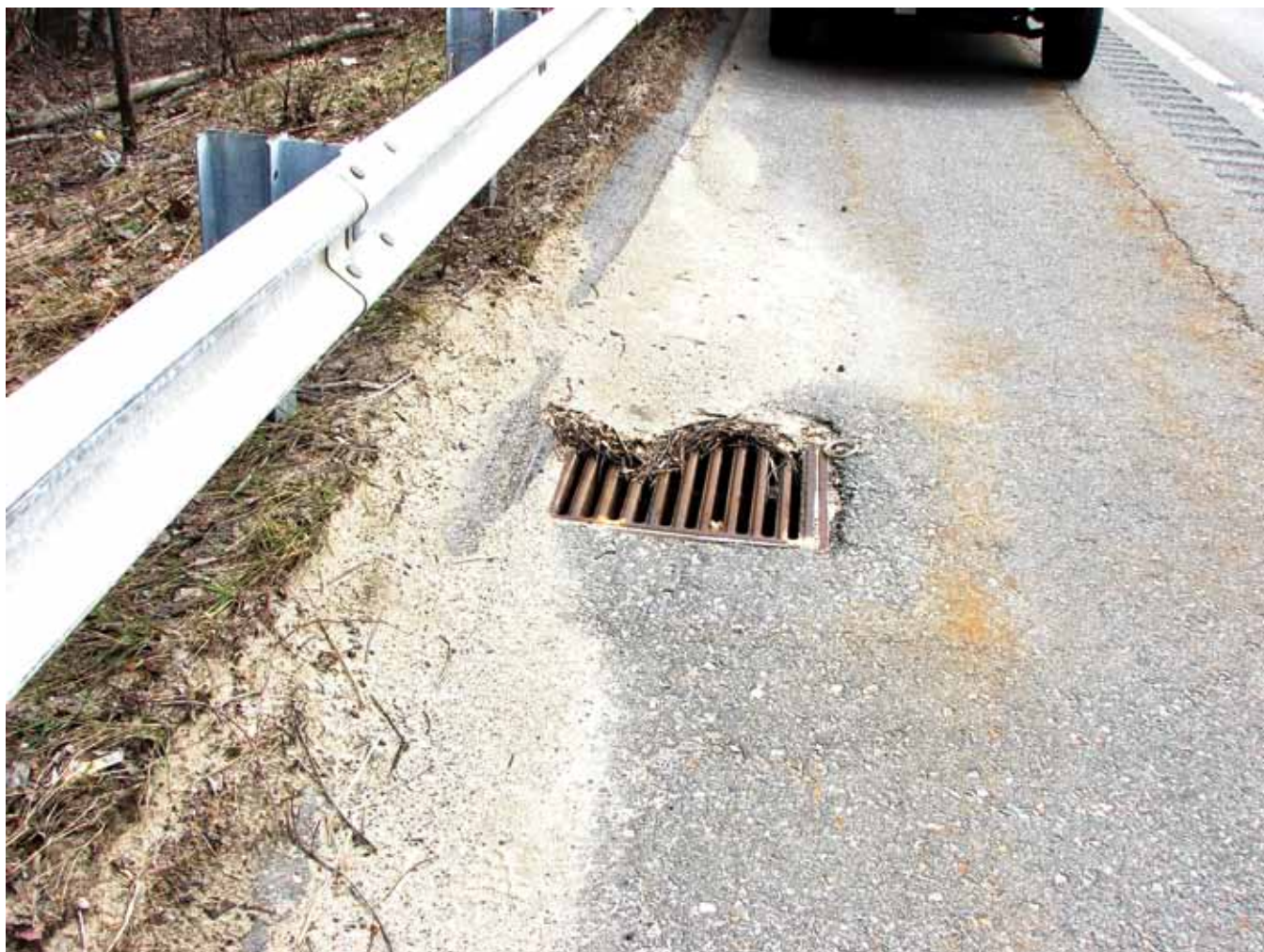
Figure 5. Sand debris around a catch basin on Route 2 in Littleton, Massachusetts, that may divert highway runoff to the next downgradient catch basin.
