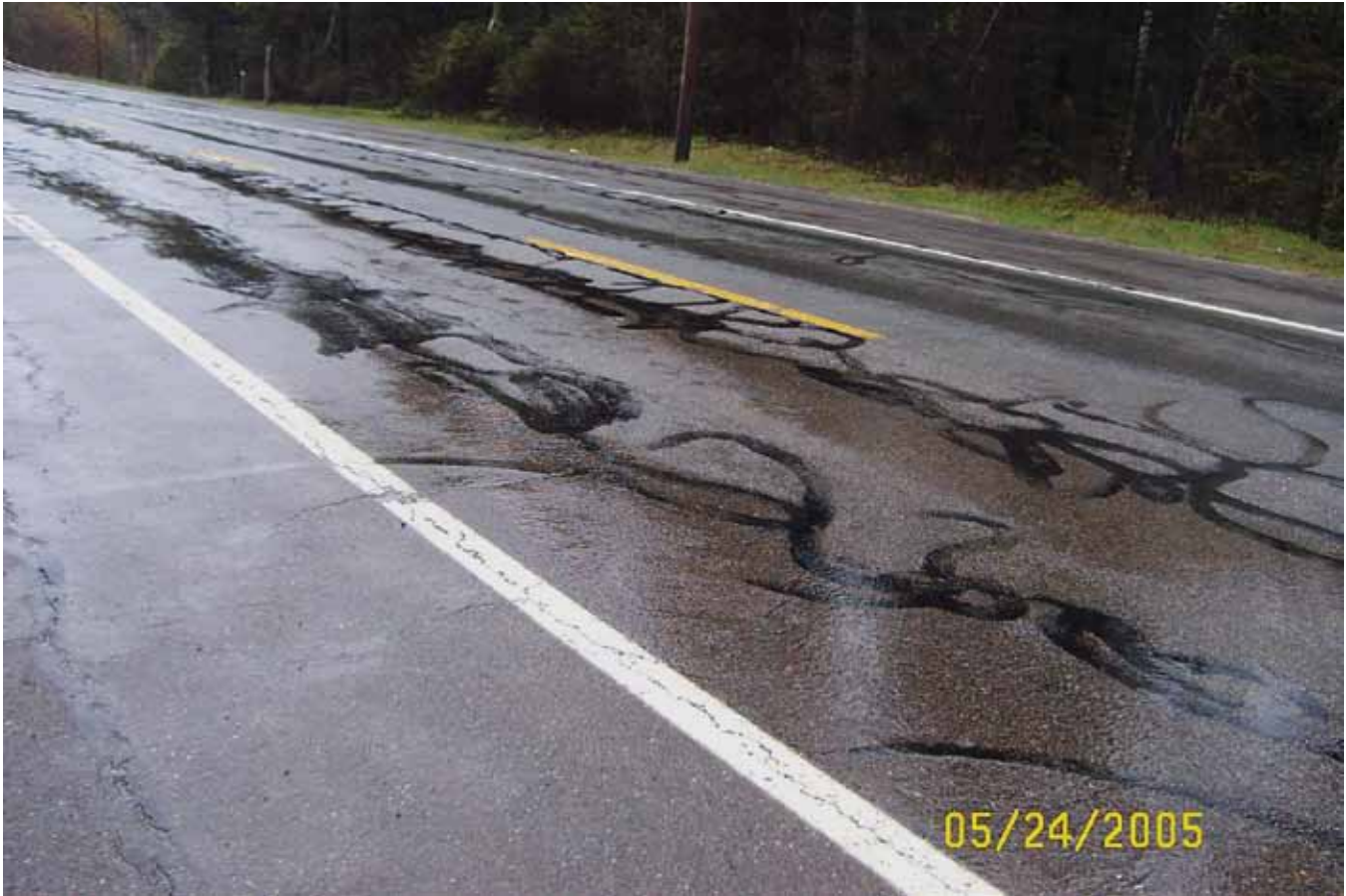
Figure 17. Ruts on the roadway surface running parallel with the road that often caused small flows to bypass the catch basin at the secondary highway-monitoring station on Route 119 in Ashburnham, Massachusetts.
