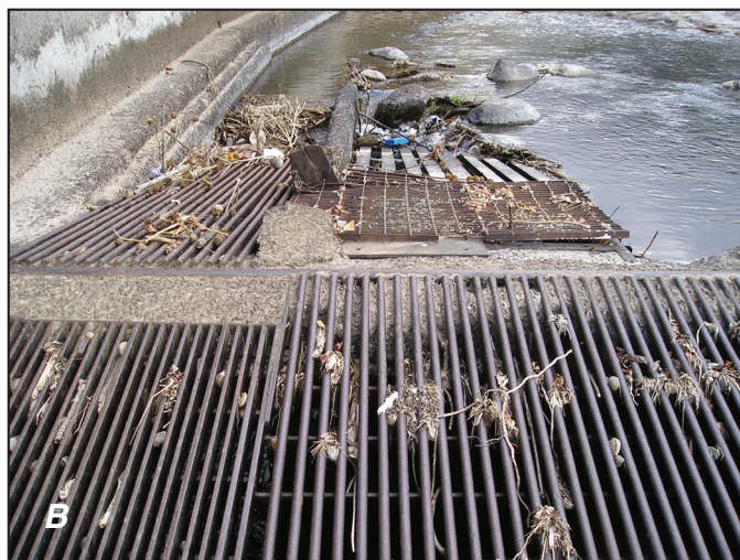
Figure A11. Photographs of Spreckels Ditch diversion intake on the south side of 'Iao Stream near an altitude of 250 feet, Maui, Hawai'i. A , Diversion intake just upstream of concrete chute (June 6, 2006). B , Closeup of parts of intake grate (June 6, 2006).
