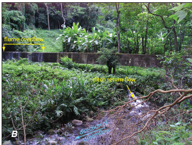
Figure 44. Photographs of overflowing flumes discharging water originating from one stream into another stream, Maui, Hawai'i. A , Spreckels Ditch overflowing into 'Īao Stream near an altitude of 220 feet (September 19, 2007). B , Waihe'e Ditch overflowing into South Waiehu Stream near an altitude of 550 feet (July 17, 2006).
