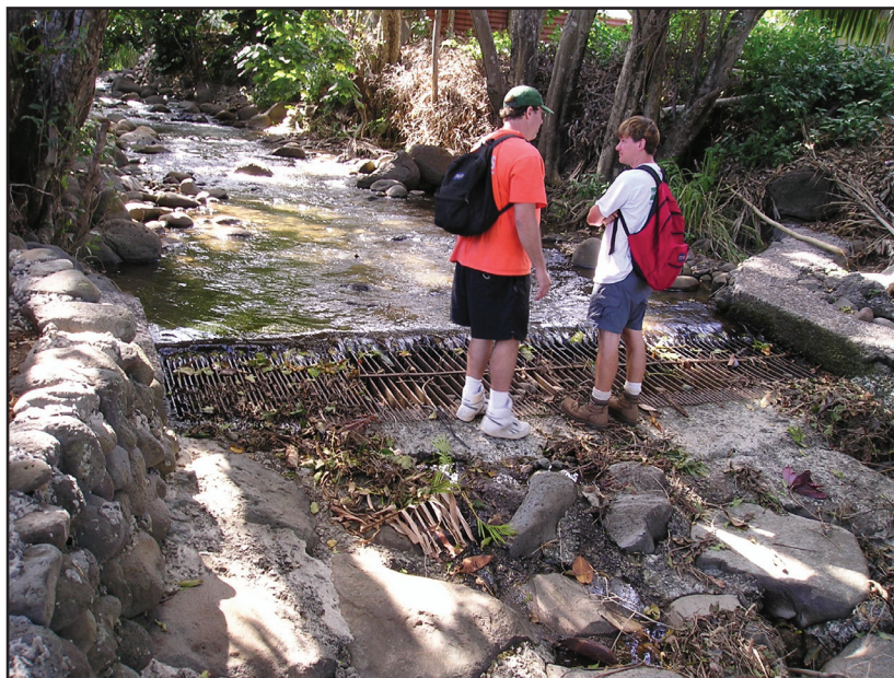
Figure A16. Photograph of diversion intake for the Reservoir 6 Ditch near an altitude of 410 feet, Waikapū Stream, Maui, Hawai'i (March 17, 2005).
