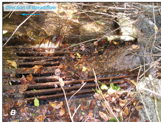
Figure A13. Photographs of Everett Ditch diversion intake near an altitude of 900 feet, Waikapū Stream, Maui, Hawai'i (August 23, 2006). A , Diversion intake near the left side (viewed downstream) of the channel being cleared of debris. B , Intake grate cleared of debris.
