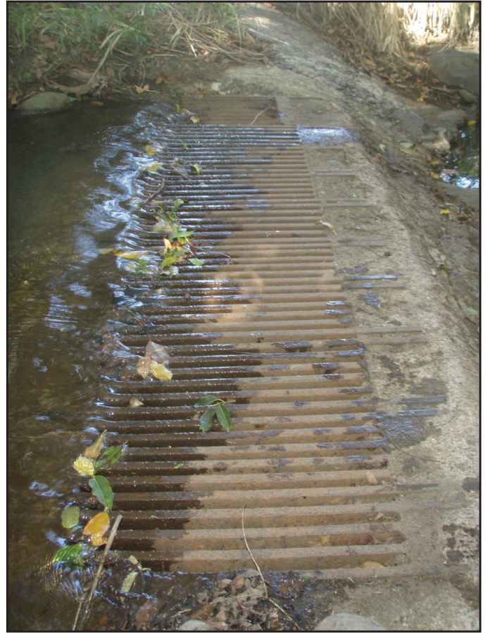
Figure A15. Photograph of diversion intake for Waihe'e Ditch near an altitude of 440 feet, Waikapū Stream, Maui, Hawai'i (October 22, 2008).
