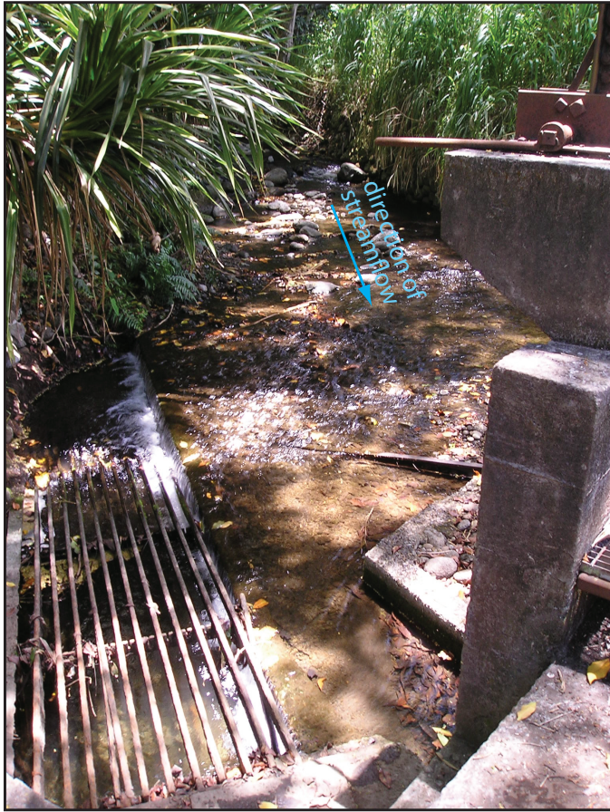
Figure A8. Photograph of Spreckels Ditch diversion intake on the south side of South Waiehu Stream near an altitude of 270 feet, Maui, Hawai'i (July 27, 2006).
