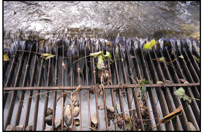
Figure ES2. Photograph of a typical diversion intake that commonly stretches across the entire low-flow channel of a stream (Reservoir 6 intake on Waikapū Stream, Maui, Hawai‘i, March 17, 2005). Water that enters the intake grate drains into a collection sump and flows by gravity into a ditch system.
