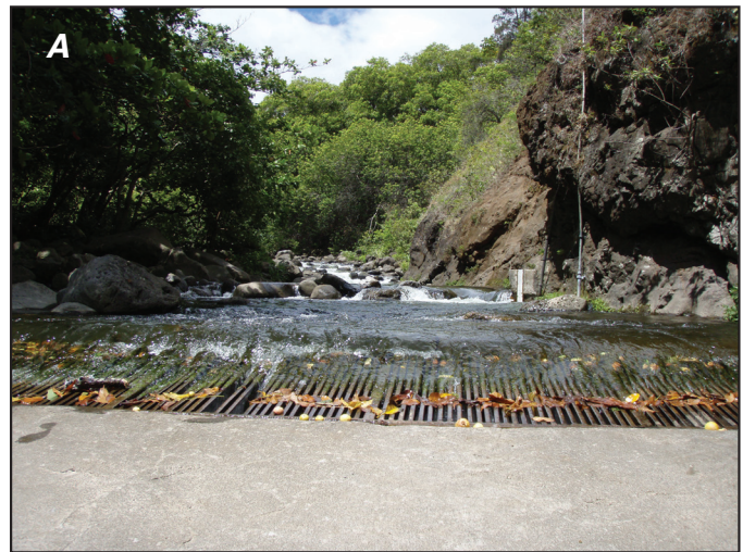
Figure A8. Photograph of Spreckels Ditch diversion intake on the south side of South Waiehu Stream near an altitude of 270 feet, Maui, Hawai'i (July 27, 2006).
