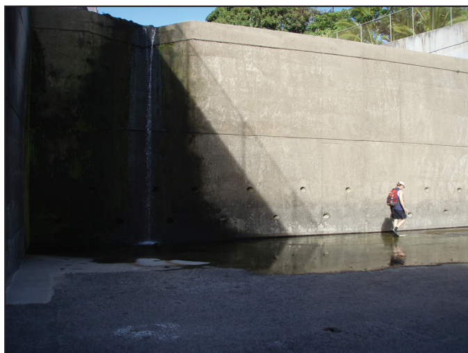
Figure 18. Photograph of vertical drop structure in concrete-lined channel near an altitude of 220 feet, 'Īao Stream, Maui, Hawai'i (August 13, 2008).
