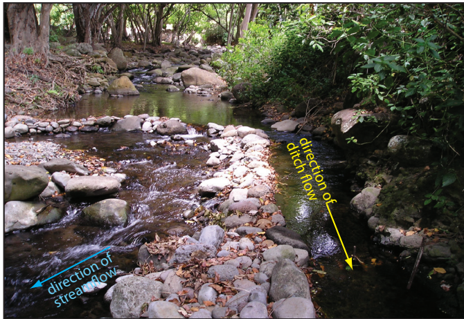
Figure A14. Photograph of diversion intake for private 'auwai (ditch) on the north side of Waikapū Stream near an altitude of 560 feet, Maui, Hawai'i (June 9, 2006).
