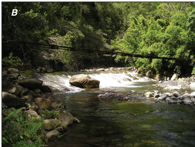
Figure A4. Photographs of dam structure for Spreckels Ditch diversion intake near an altitude of 400 feet, Waihe'e River, Maui, Hawai'i. A , Typical dry weather diverted condition (August 7, 2006). B , During ditch maintenance period when water was temporarily restored to Waihe'e River (June 8, 2006).
