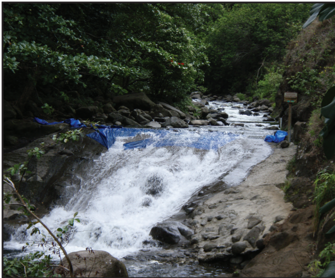
Figure 46. Photograph of partially covered (with blue tarp) diversion intake common to the 'Īao-Mānania and 'Īao-Waikapū Ditches near an altitude of 780 feet, 'Īao Stream, Maui, Hawai'i (July 30, 2007).
