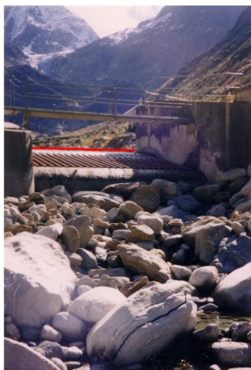
Figure 5. The water intake at the Tyrolean weir in the Pitzbach (photo courtesy of TIWAG). The PBIS sensors were mounted at the upstream end of the weir (location marked with red line).
