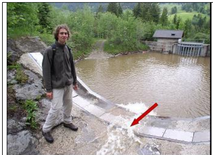
Figure 3. The PBIS array for measuring bedload transport in the Erlenbach is mounted underneath steel plates at the crest of a large check dam. The red arrow points to the steel plate of sensor no. 3.
