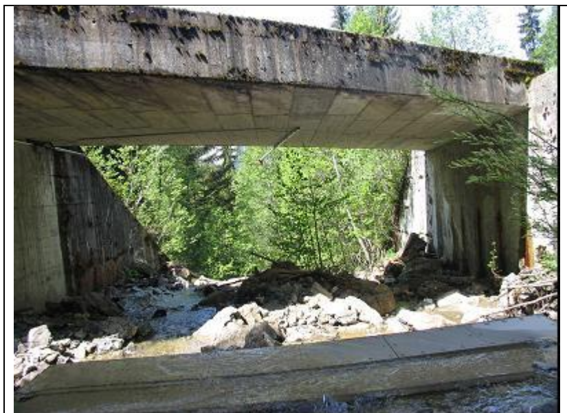
Figure 7. A PBIS array mounted in the Erlenbach at a check dam ("upstream row") about 500 m upstream of the retention basin. A second array is installed at a check dam 14 m downstream of the check dam shown here.
