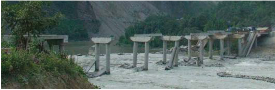
Figure 7. Damage scenario of the 10-span bridge under construction during the earthquake.
