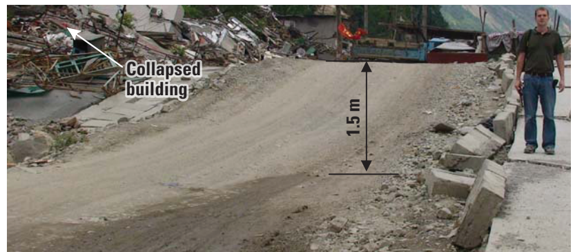
Figure 3. Surface rupture along the Old Highway near the collapsed building.
