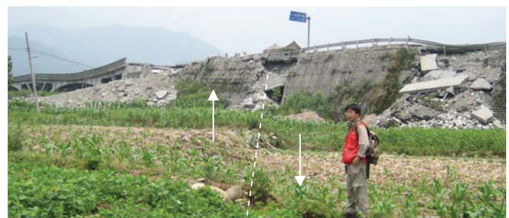
Figure 4. Surface rupture at Xiaoyudong Bridge site ( http://www.uky.edu/KGS/geologichazards/Sichuan_Earthquake.pdf ).
