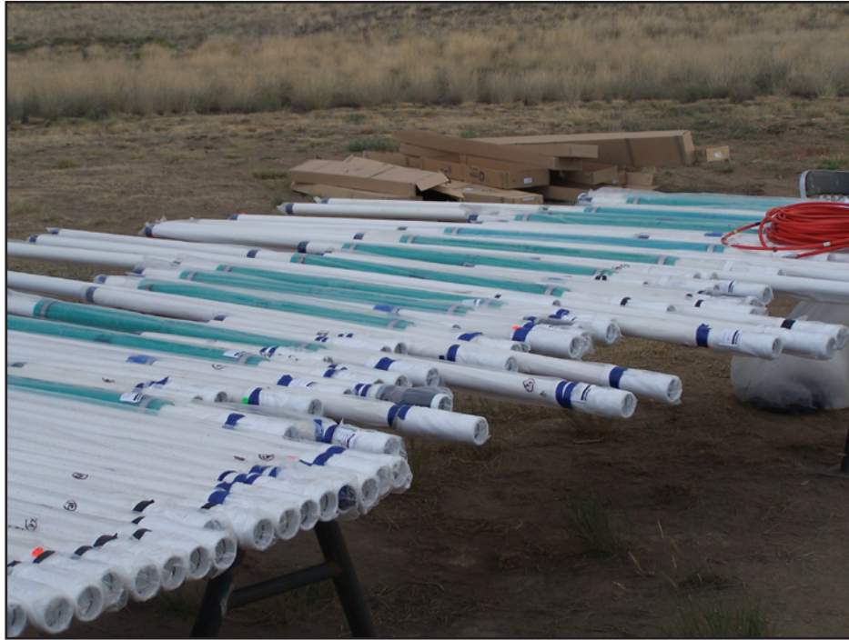
Figure 5. Pre-assembly of the components during the layout phase of Multilevel Monitoring System installation, Idaho National Laboratory, Idaho, 2007–08.
