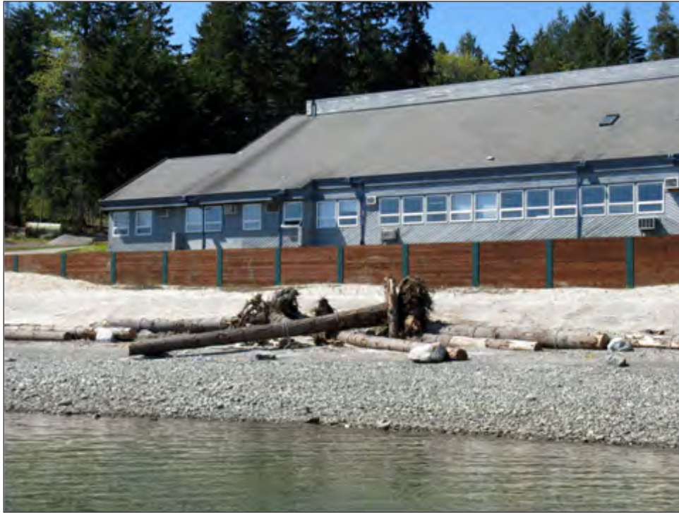
Bank stabilization project in front of building, showing vertical pile wall, recently planted and regraded slope (covered with mesh), and large anchored logs.
