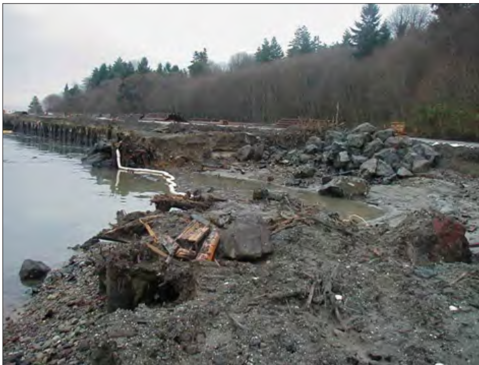
Initial excavation of historic fill and debris on western portion of the site (Source: Eric Nelson, U.S. Army Corps of Engineers.)
