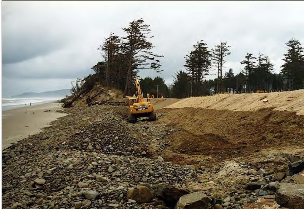
**Figure 6.** Construction of the cobble berm and artificial foredune in Cape Lookout State Park during the fall of 2000. A continuation of the old dune ridge is seen in the background, which had previously extended past this area of erosion.
