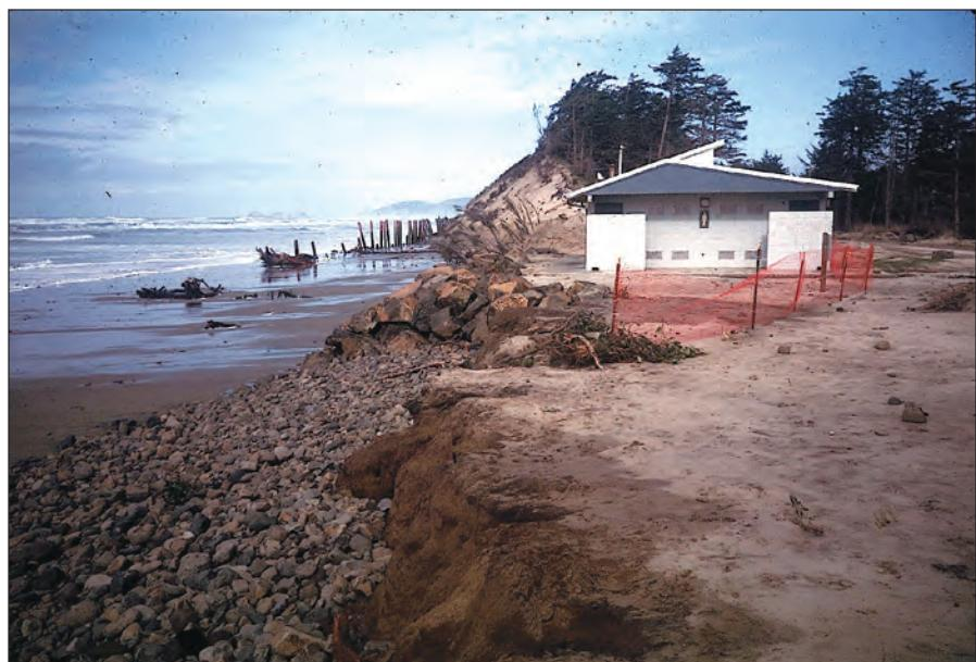
**Figure 4.** Erosion of Cape Lookout State Park, photographed during the 1997–98 El Niño. The remnants of the high dune ridge and a failed log seawall are seen in the background. Riprap temporarily protected the bathrooms, but they were removed after having been damaged the following winter when the March 1999 storm breached this area and washed through the campground (Allan and Komar, 2004).
