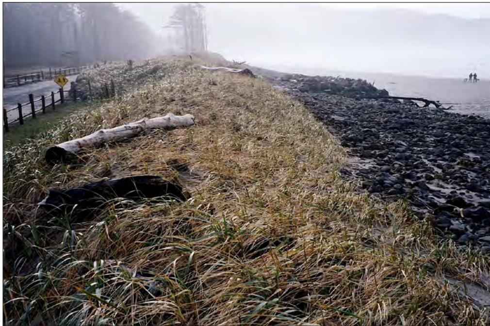
**Figure 7.** Completed cobble berm and foredune, having been overtopped by a winter storm along the stretch that had not been constructed to the designed elevations. The riprap that previously had protected the bathrooms (fig. 4) can be seen in the background.
