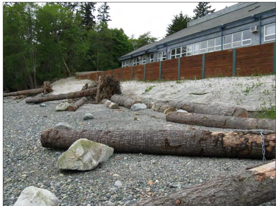
**Figure 9.** Logs at the back of a gravel beach on the shore of Puget Sound, placed to protect the property from high tides and waves.
