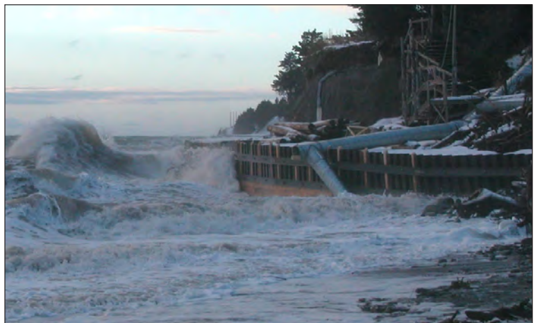
Figure 1. Seawalls impact nearshore hydrodynamics in many ways, including wave reflection. Photo Credit Carl Schoch (Homer, Alaska).
