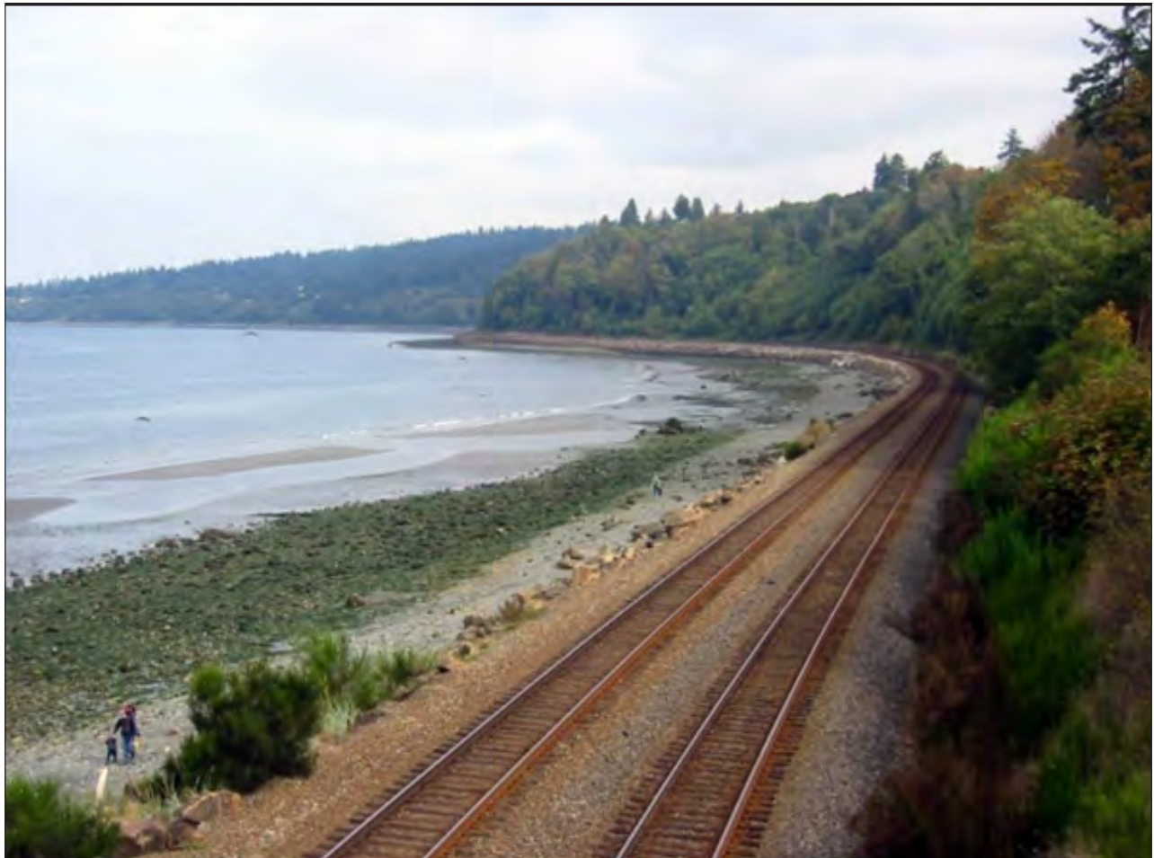
Figure 6. Railroad along the shoreline between Seattle and Everett. The seawall was constructed in the early 1900s to protect the railroad, which had been built on the beach below the high bluffs. The upper beach is buried by the railroad grade. This photograph was taken at an extreme low tide; a normal high tide would extend to the seawall, leaving no beach exposed.
