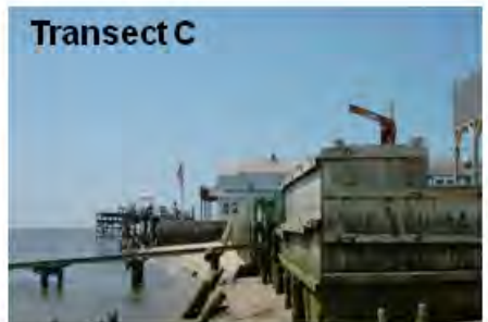
Figure 3. Complex platform configuration and differences in beach width resulting from incremental bulkhead construction.
