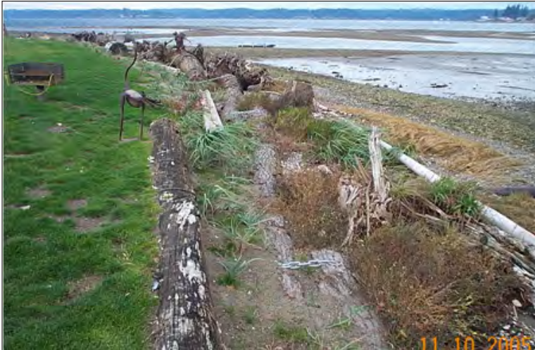
Figure 5. Mercer large wood placement, Key Peninsula, Washington.
