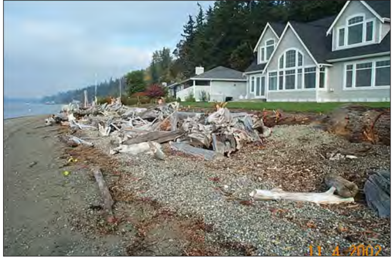
Figure 3. Turnbull large wood placement, Fox Island, Washington.
