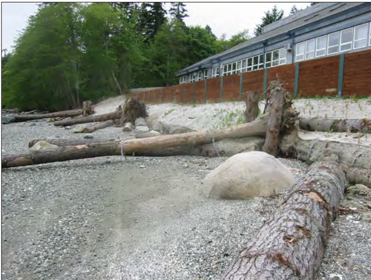
Figure 6. Suquamish Tribal Natural Resources large wood and bank resloping, Agate Pass, Washington
