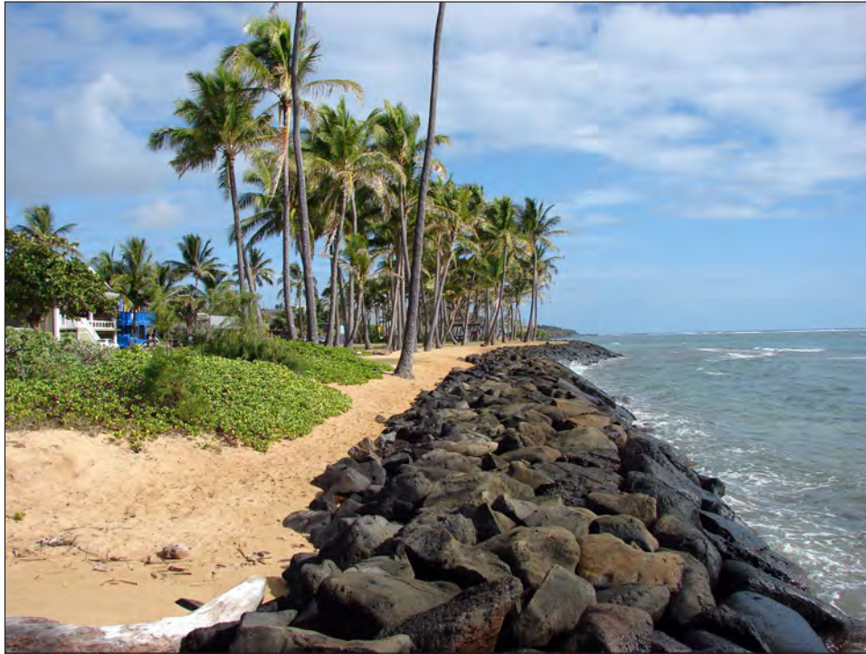
Figure 4. Coastal armoring along the central coast of the Island of Kauai, Hawaii resulting in the loss of the fronting beach due to passive erosion and source sediment impoundment.
