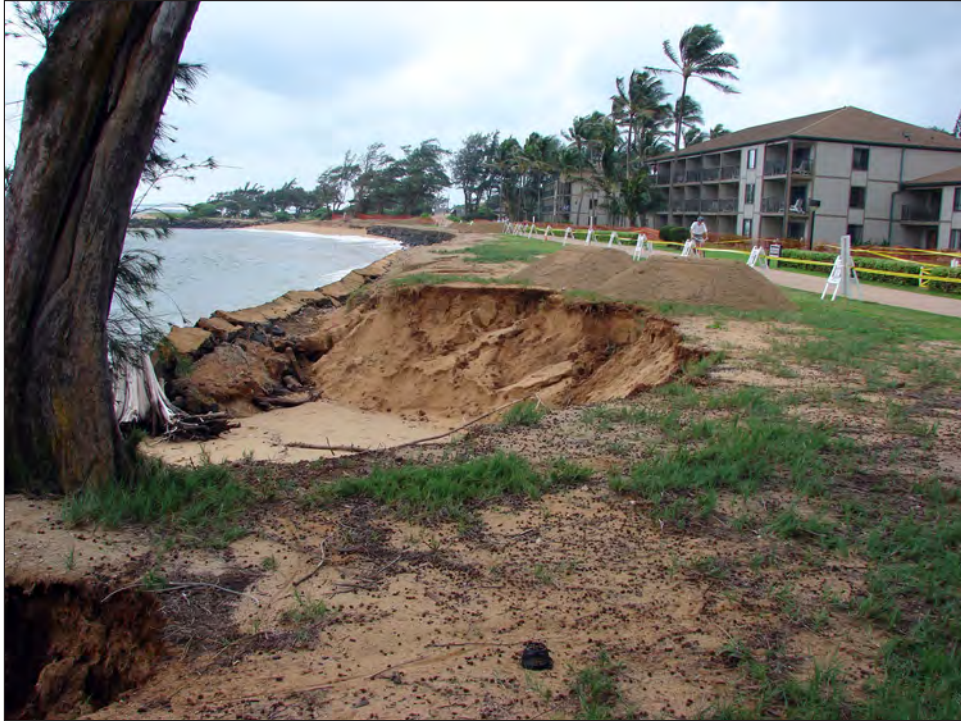
Figure 8. End scour or flanking erosion at a seawall along the east coast of the Island of Kauai, Hawaii.
