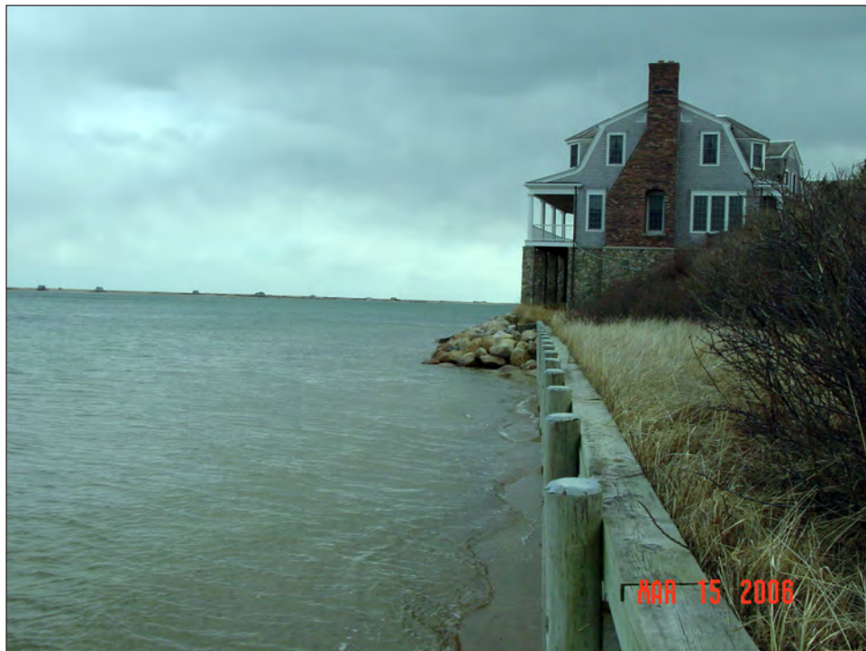
Figure 9. Depiction of the extent of placement loss of beach and marine habitat by comparing the extent of loss due to a revetment vs. a bulkhead.
