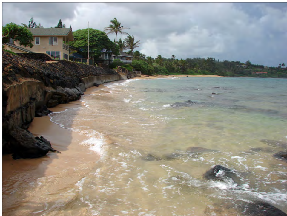
Figure 6. The loss of beach and thus public lateral beach access due to shoreline armoring and chronic erosion along the east coast of the Island of Kauai, Hawaii. Note the sandy beach in the background where no coastal armoring exists.
