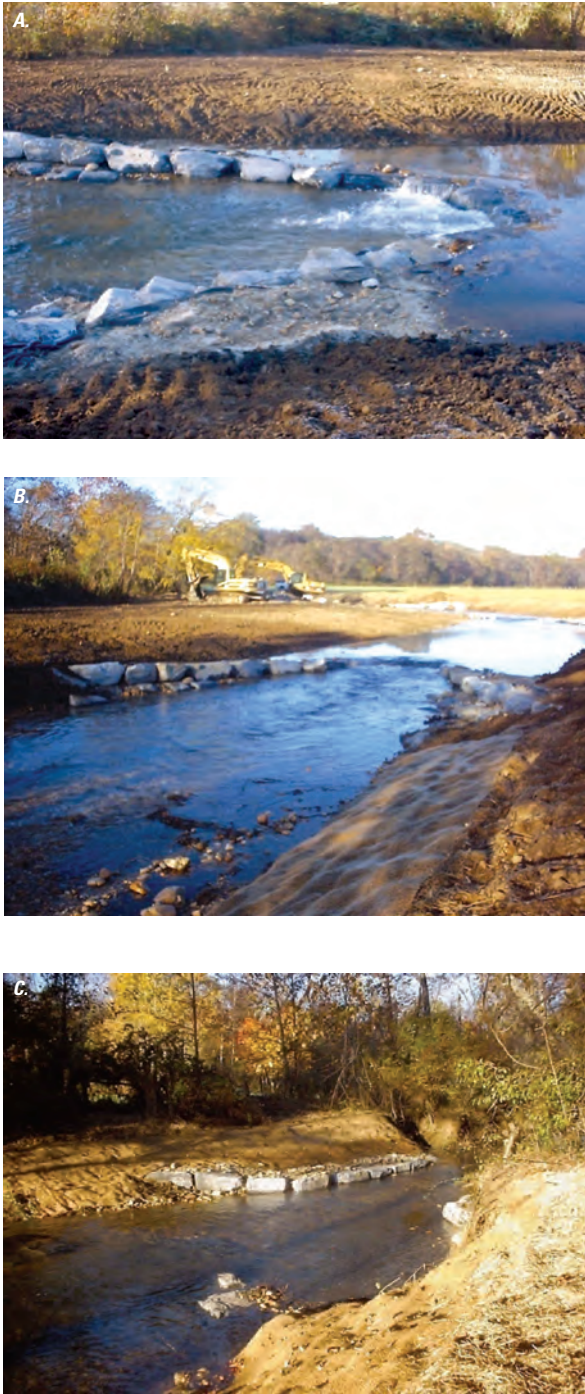
Figure 9. The restored reach upstream from the streamgaging station at Pauls Creek near Pine Ridge, North Carolina, showing (A) typical rock vane structure installed in the stream channel upstream from the streamgaging station, (B) channel-stabilization work in progress on November 4, 2005, and (C) typical bank-stabilizing structure installed in the stream channel upstream from the streamgaging station.
