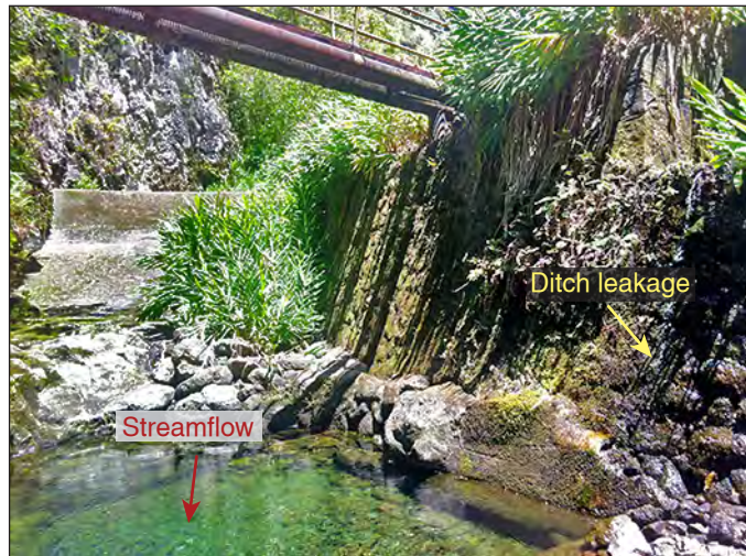
Figure 10. Photograph showing leakage from Honokōhau Ditch downstream from the diversion dam on Kapāloa Stream, Maui, Hawai'i, during the seepage run on July 25, 2012.
