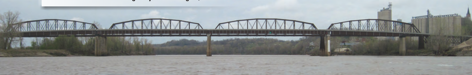
Structure G0069 on State Highway 240 at Glasgow, Missouri.
