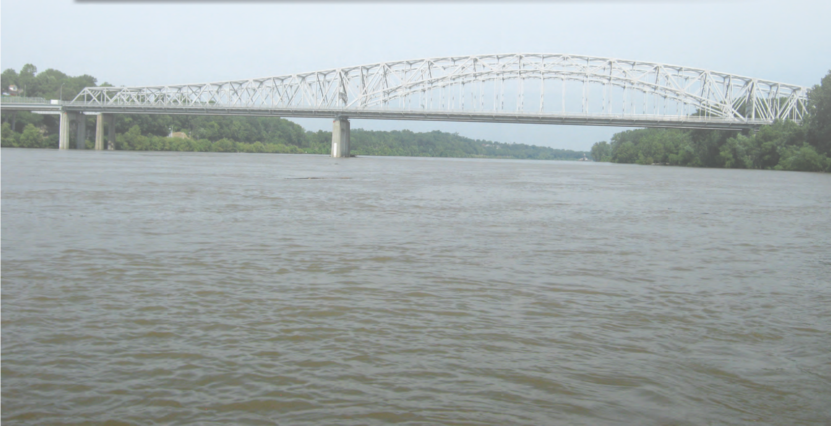
Structures L0550 and A4497 on U.S. Highway 54 at Jefferson City, Missouri.
