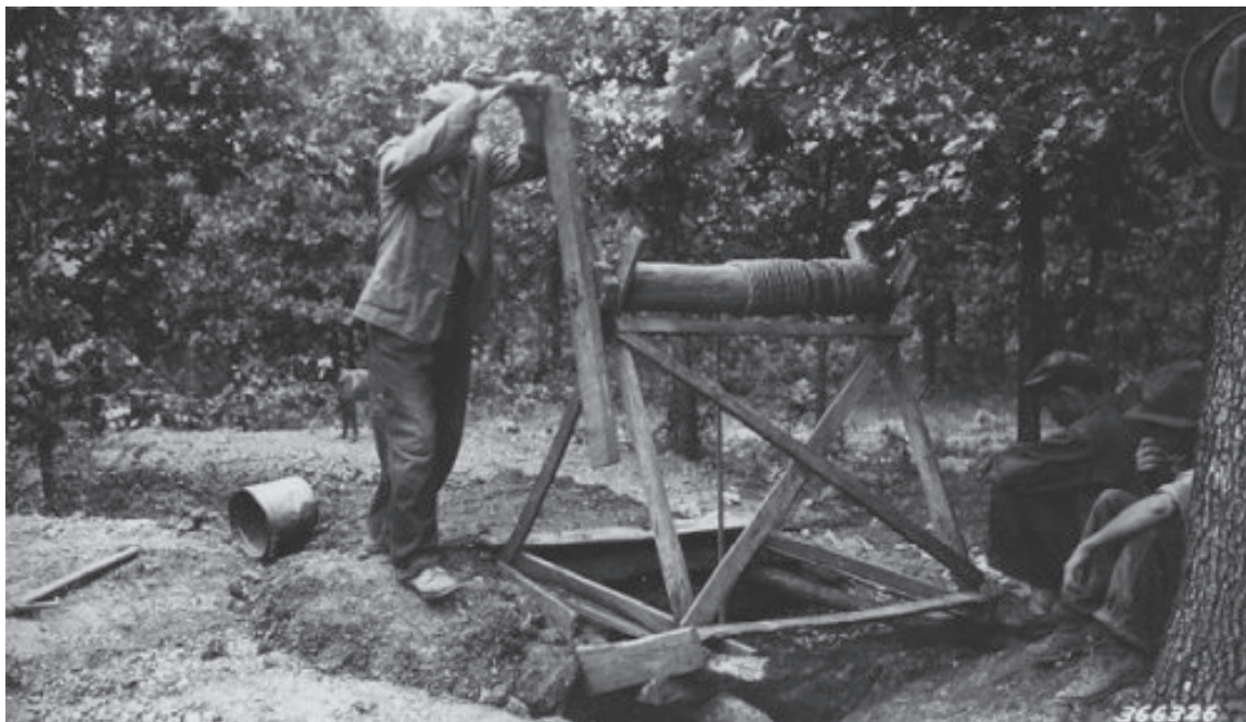
A. Miner operating windlass to hoist barite ore to the surface
