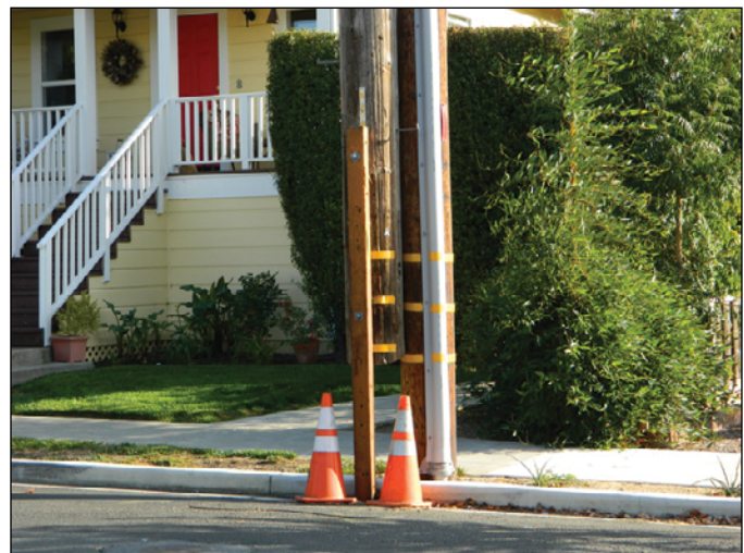
Figure 19. Photographs showing repair dependence between telecommunications and electrical power poles. After the 2014 South Napa, California, earthquake, a wooden telecommunications pole was observed to have been quickly repaired with a 2×6 support and tied to the adjacent power pole. A , Photograph of full pole with repair. B , Close-up view of wooden support repair. Photographs by A. Tang, L&T Consultant, October 20, 2015, used with permission.
