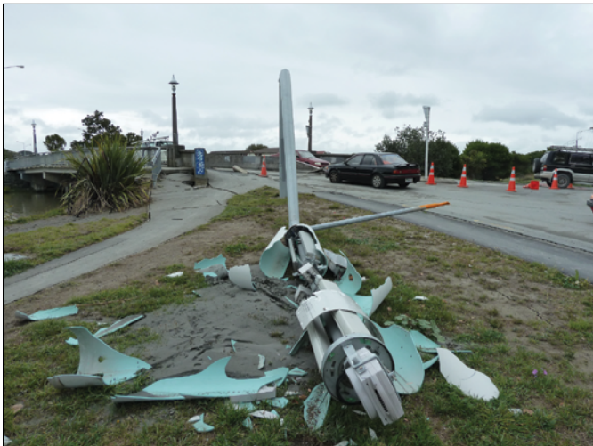
Figure 6. Photograph showing utility pole damage to a cellular site after the 2011 Christchurch, New Zealand, earthquake. The pole split along a fold seam midway up the pole; the head load is thought to be the issue (Wes Bonney, written commun., March 26, 2021). Photograph from Wes Bonney, Vodafone, New Zealand, February 22, 2011, used with permission.
