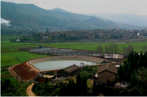
Figure 4. Exploitation and utilization of Pijiazhai karst spring (flow of 1.0 to 1.9 m 3 /s) for water supply and irrigation in Luxi Basin, Yunnan Province, China. It was exploited and utilized by installation of a grout curtain in order to concentrate groundwater discharge.
