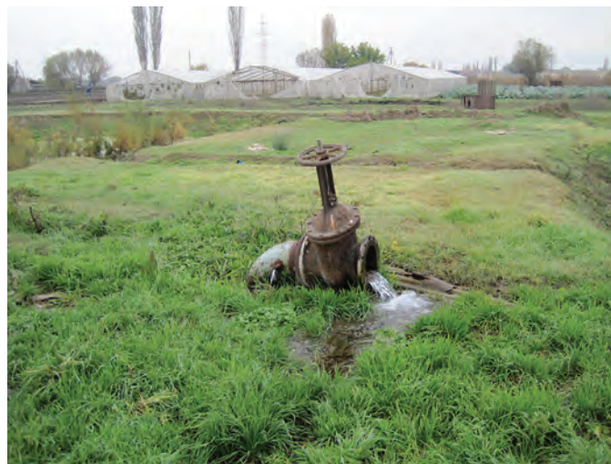
Figure 17. An abandoned well flowing water to the land surface in November 2015 in the Ararat Basin in Armenia.
