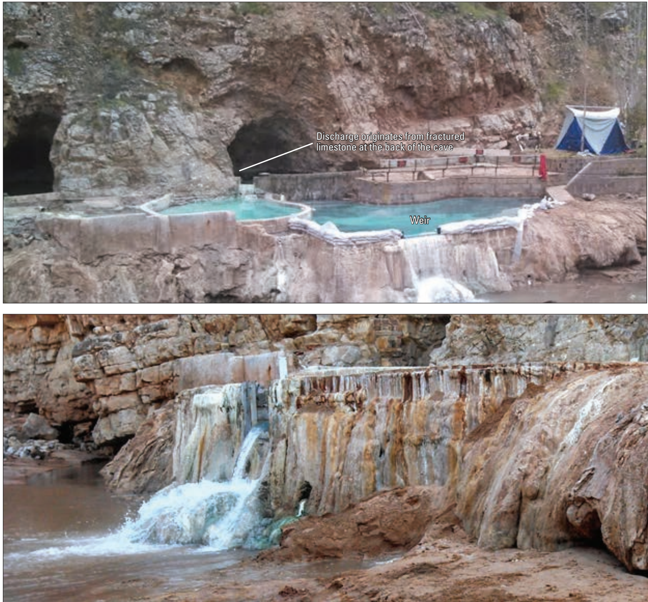
Figure 13. Man-made pools below the grotto spring (PTGS) and the weir used to monitor discharge during the three interference tests at Pah Tempe Springs, Washington County, Utah. Note the massive travertine deposits, formed by precipitation of calcium carbonate from the springwater.
