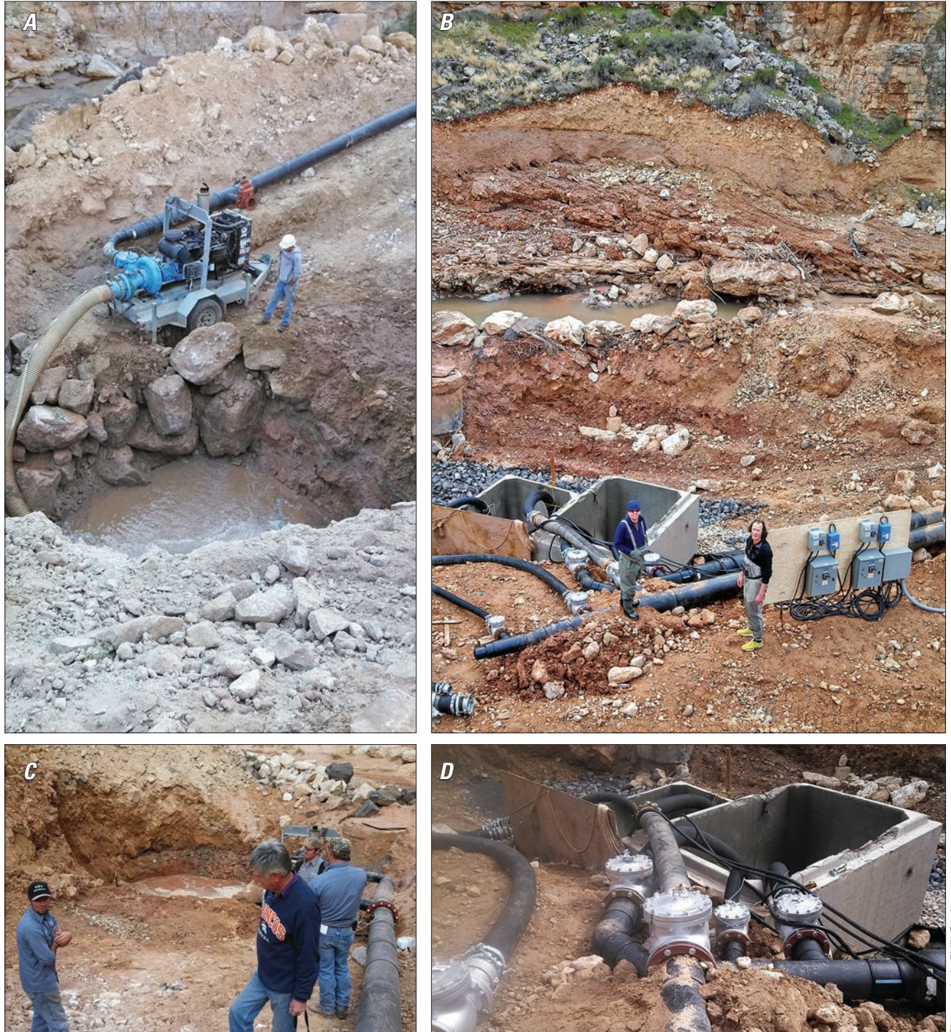
Figure 4. Original sump structure (A and C, November 2013) and improved sump structure (B and D, February and November 2014) used for pumping thermal water from the fractured carbonate-rock aquifer during Pah Tempe Springs interference testing. Upper right image B, shows concrete vaults on the north bank of the Virgin River placed on top of rip rap in the excavated sump with discharge lines from multiple submersible pumps tying into two main discharge lines (lower right in figure). Lower right image D, shows a close up of one of the manifolds where discharge lines from multiple submersible pumps join one of the main discharge lines.
