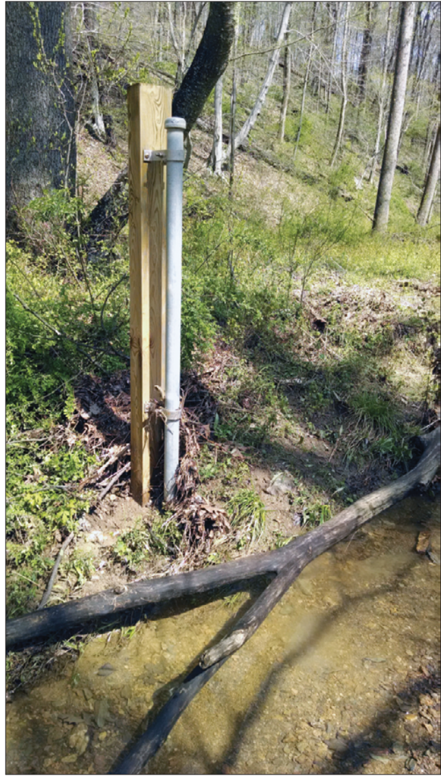
Figure 7. Crest-stage gage for obtaining high-water marks in the Tenmile Creek study reach. Photograph by Michael A. Clark, U.S. Geological Survey, May 1, 2014.
