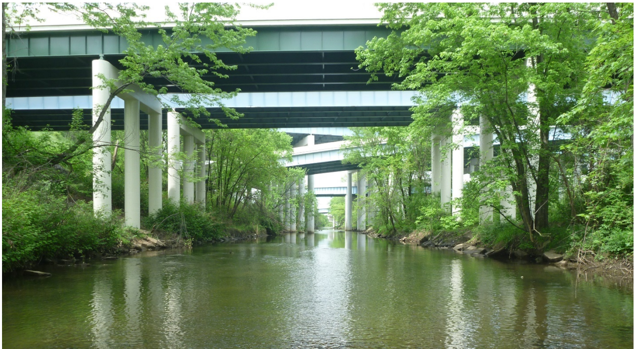
U.S. Route 30 and Interstate 77 interchange over West Branch Nimishillen Creek in Canton, Ohio.
