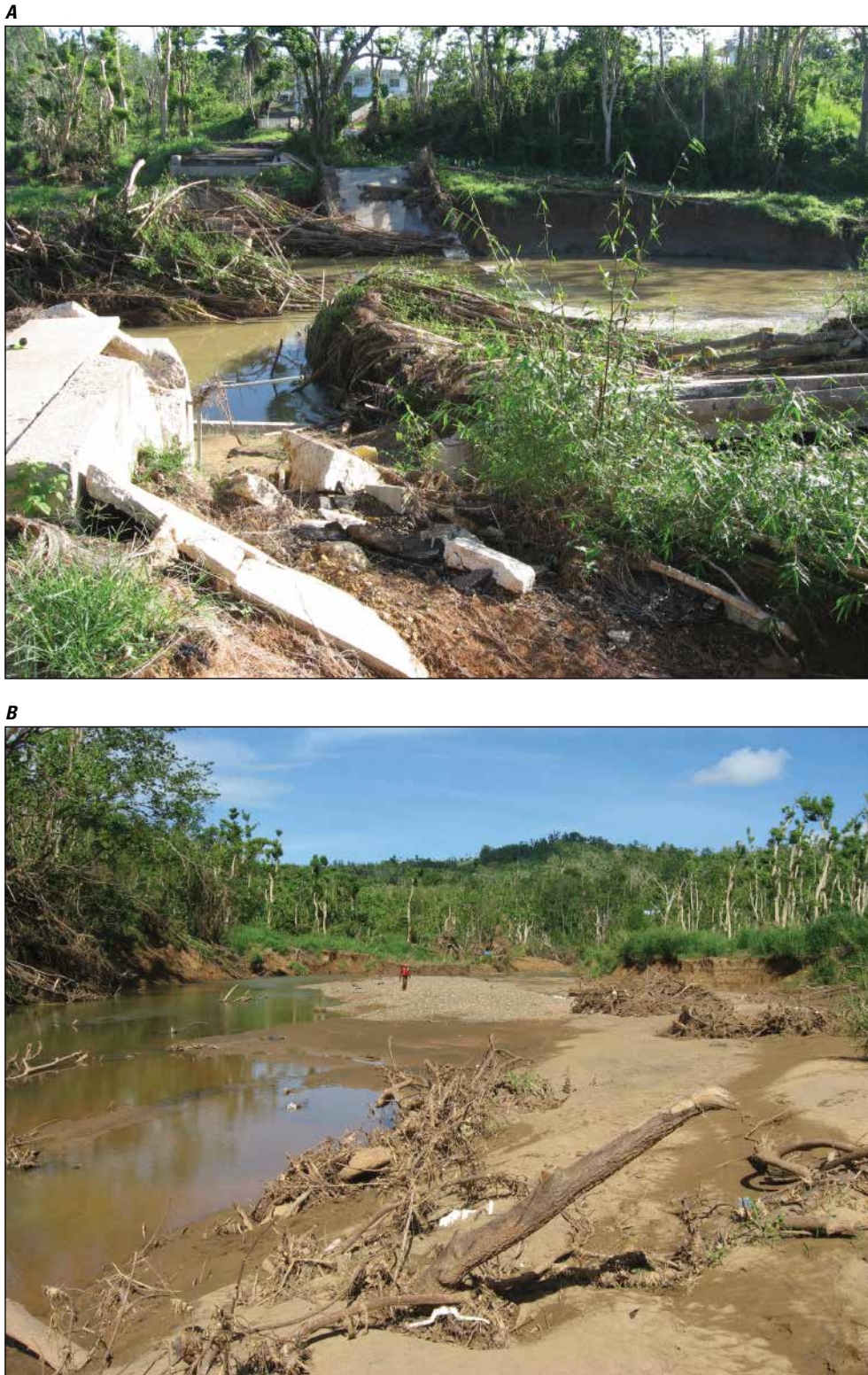
Figure 2.14. Conditions along study reach for station 50147800 Río Culebrinas at Highway 404 near Moca, November 14, 2017: A , View right to left of destroyed Highway 404 bridge where streamgage was located; B , view downstream from upstream end of study reach (600 feet downstream from streamgage). Photographs by Mark Smith, U.S. Geological Survey.
