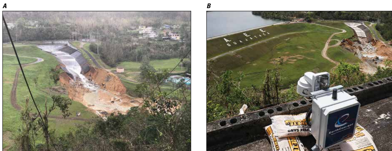
Figure 13. Photographs showing, A, the area affected by the flood of September 20, 2017 (photograph date, October 4, 2017) and, B, the high-resolution camera installed on a neighbor's rooftop near Lago Guajataca Dam for monitoring the extent of the erosion (photograph date, October 18, 2017). Photographs by John Parks, U.S. Geological Survey.
